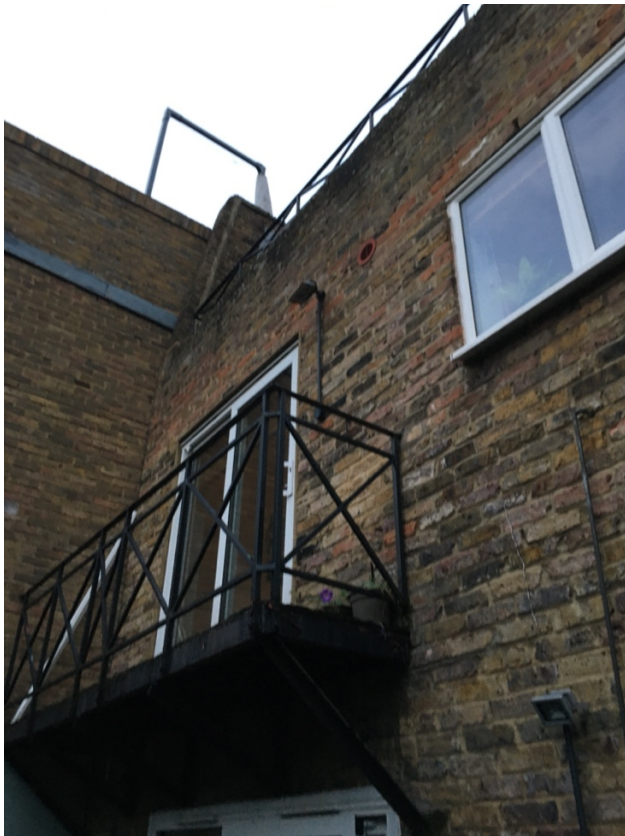
33 Camden Mews: Rear wall taken from courtyard
