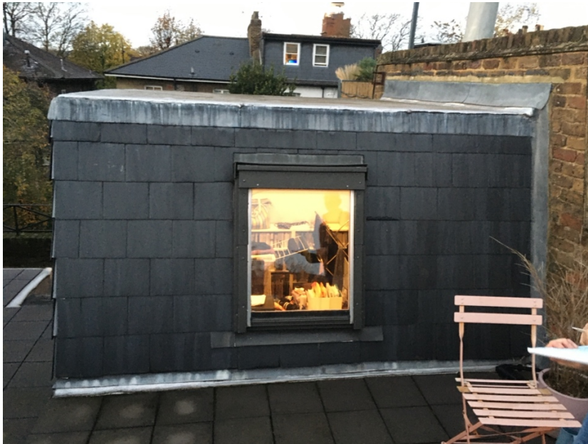
33 Camden Mews, existing roof room
