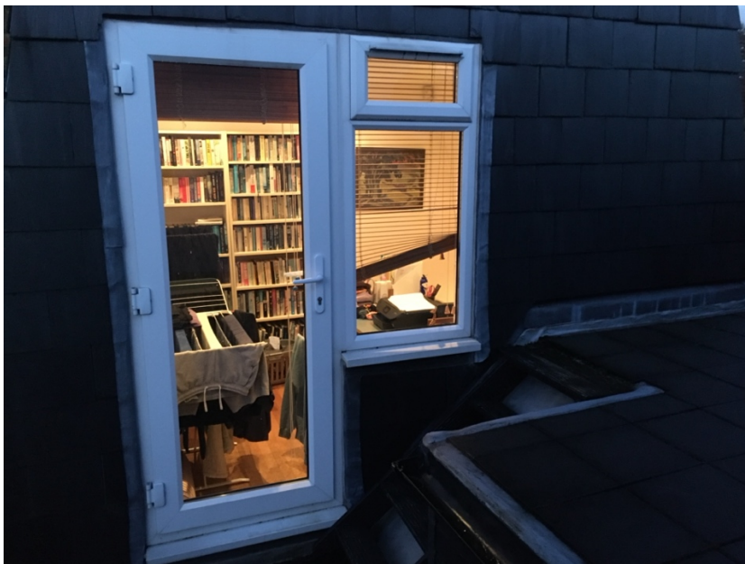
33 Camden Mews, existing door for roof terrace access
