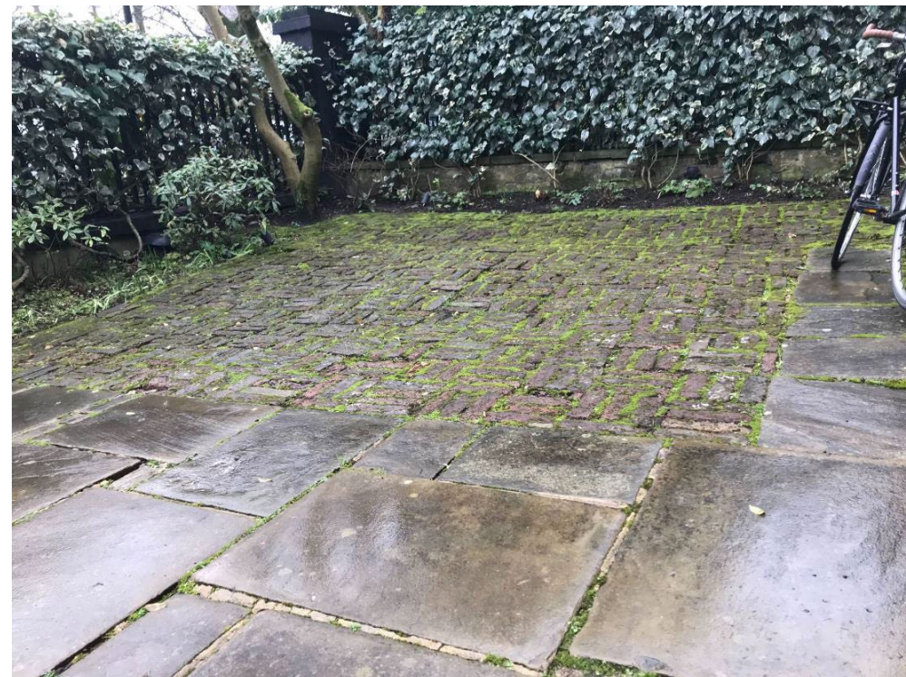
Plate 8: The southern part of the front garden. A basement area already exists beneath a portion of this.
