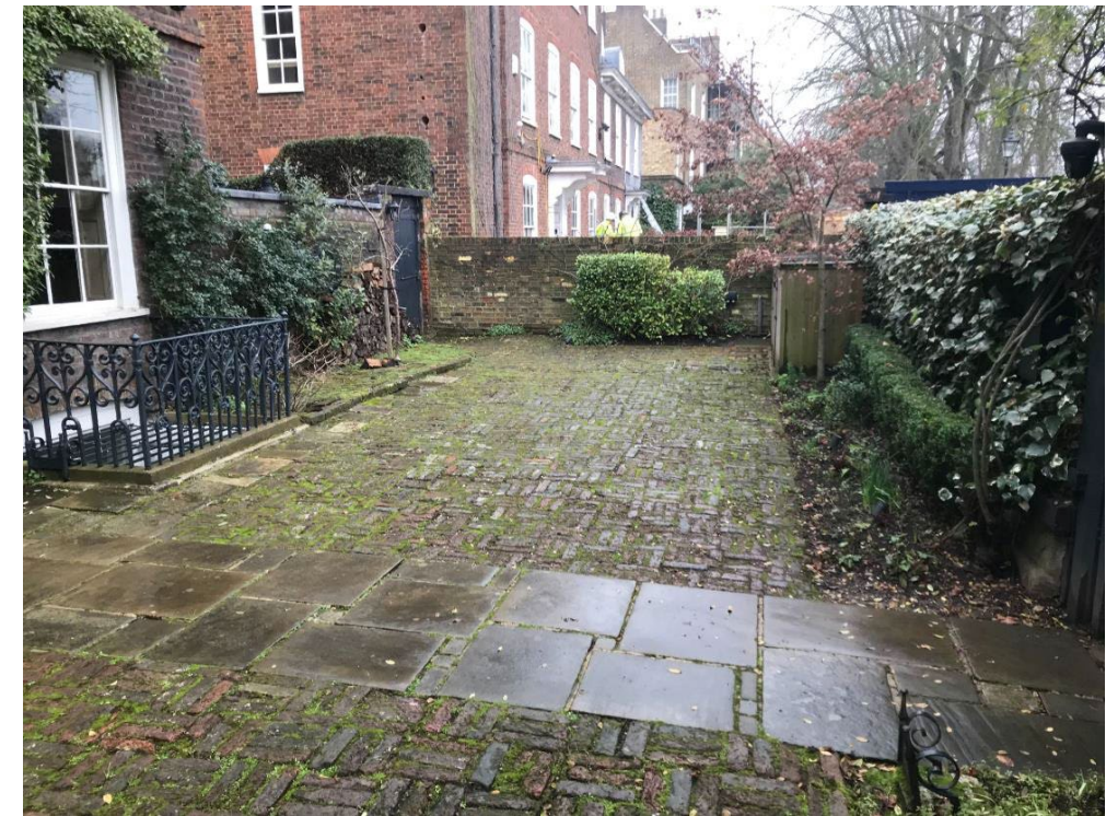
Plate 7: Front Garden of 4 The Grove. This photograph faces across the northern part of the garden. The area beyond the footpath (of slabs) is that in which a basement application is being considered
