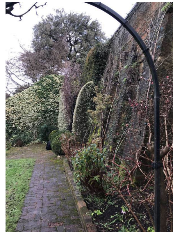
Plate 21: Photographer is facing north with the Listed (Grade II) Garden Walls, Terraces and Steps of Numbers 1-6 and Garden Arbour to Number 6 (1378982) in the right hand part of this image.
