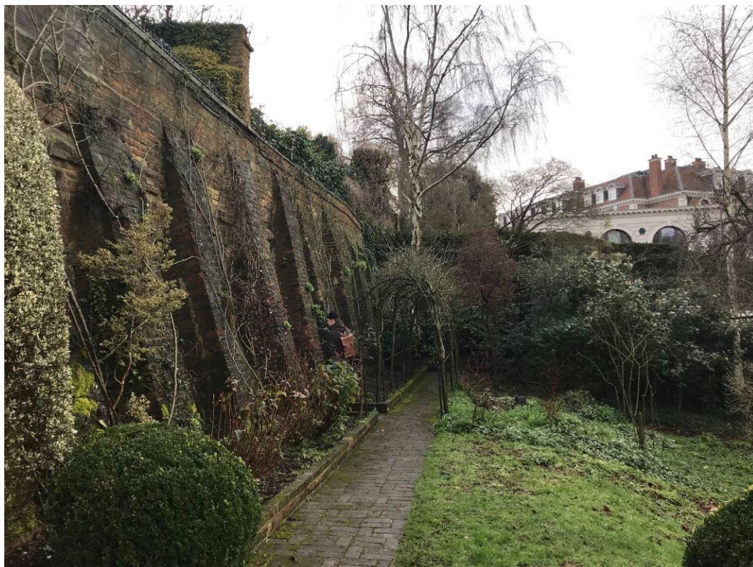
Plate 20: Photographer is facing south with the Listed (Grade II) Garden Walls, Terraces and Steps of Numbers 1-6 and Garden Arbour to Number 6 (1378982) in the left hand part of this image.
