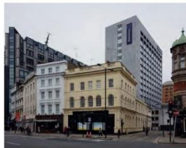
View from Coptic Street - existing
