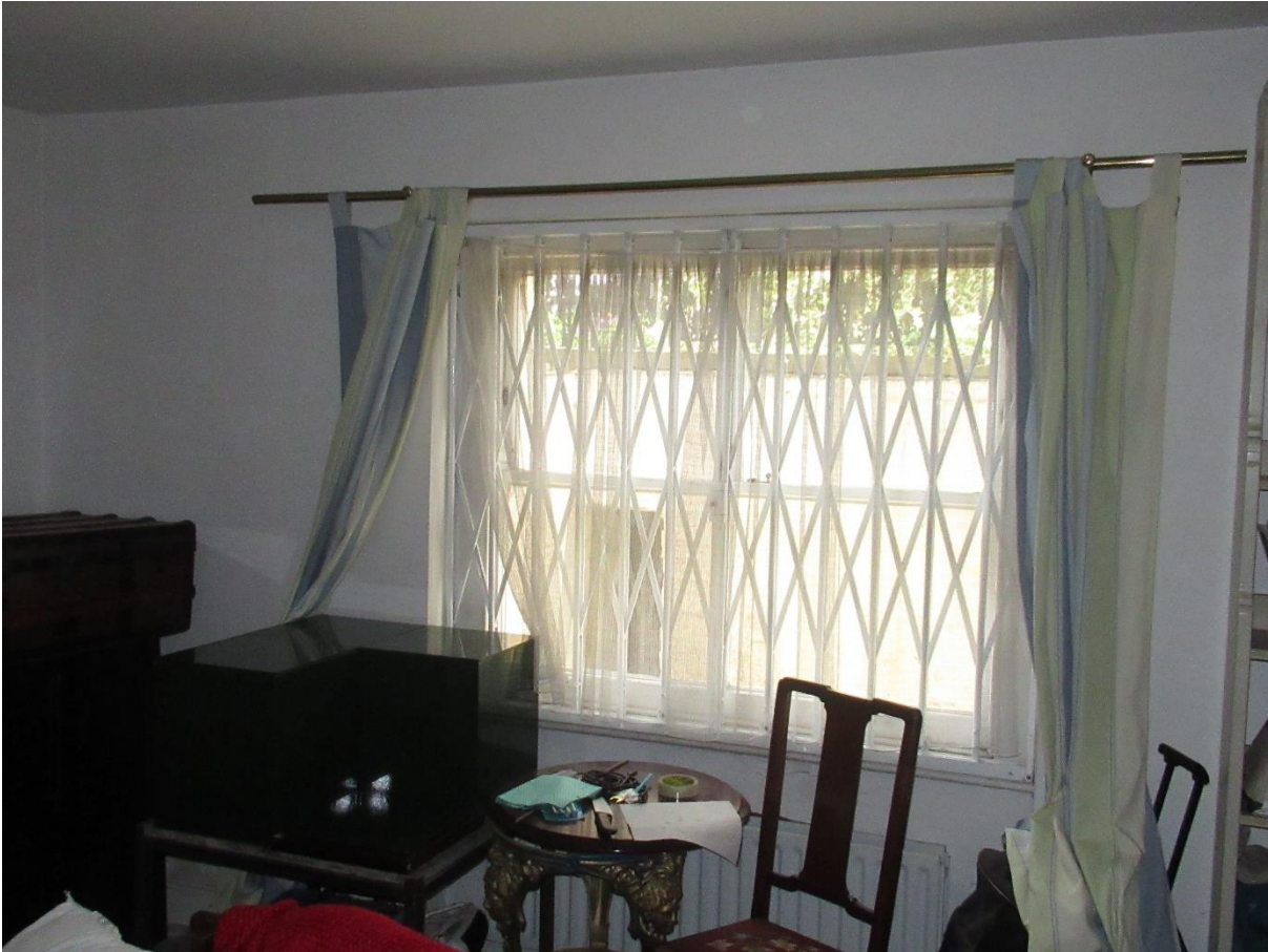
Figure 6 – Internal view of the window to the front of the building at basement floor level
