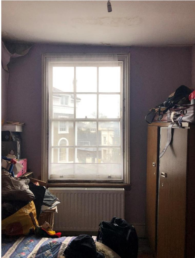
*Figure 8* – Internal view of the timber sash window in the left bedroom to the front of the building at second floor level
