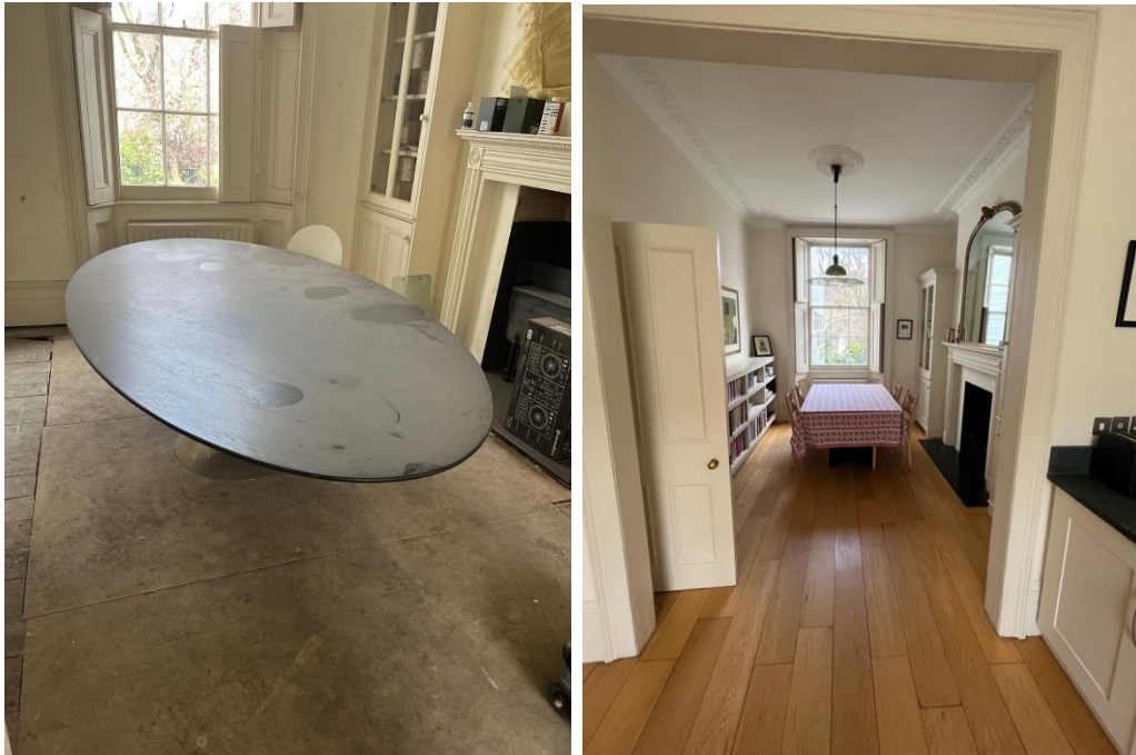
Condition of flooring remaining from previous owners showing mdf sub-floors (left image) and engineered wood on top (right).
