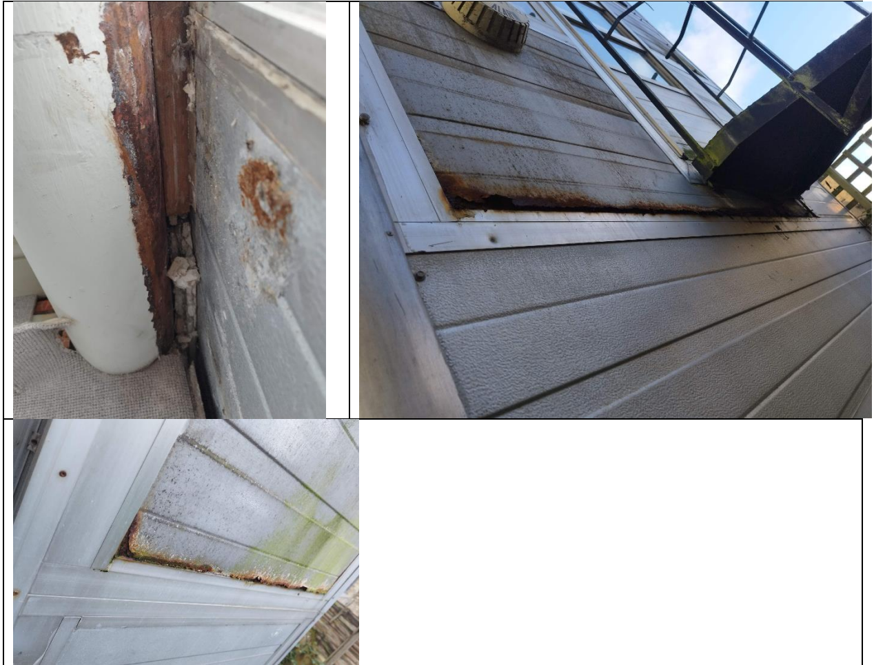
Photographs showing current condition of cladding
