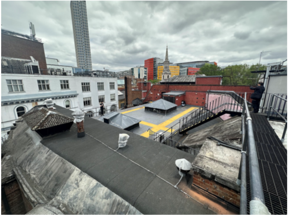
Figure 5 (above): Roof of the Phoenix Theatre
