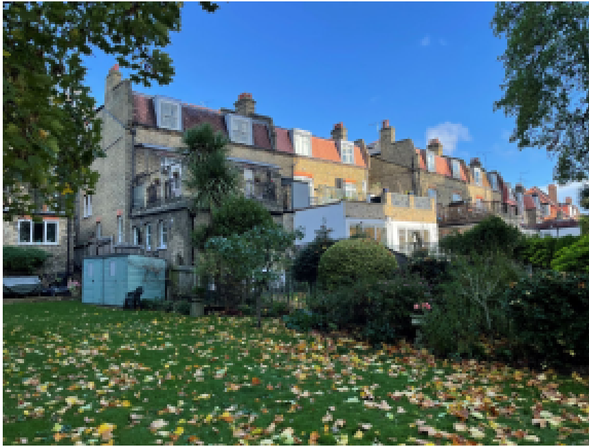
View of the rear / side boundary
