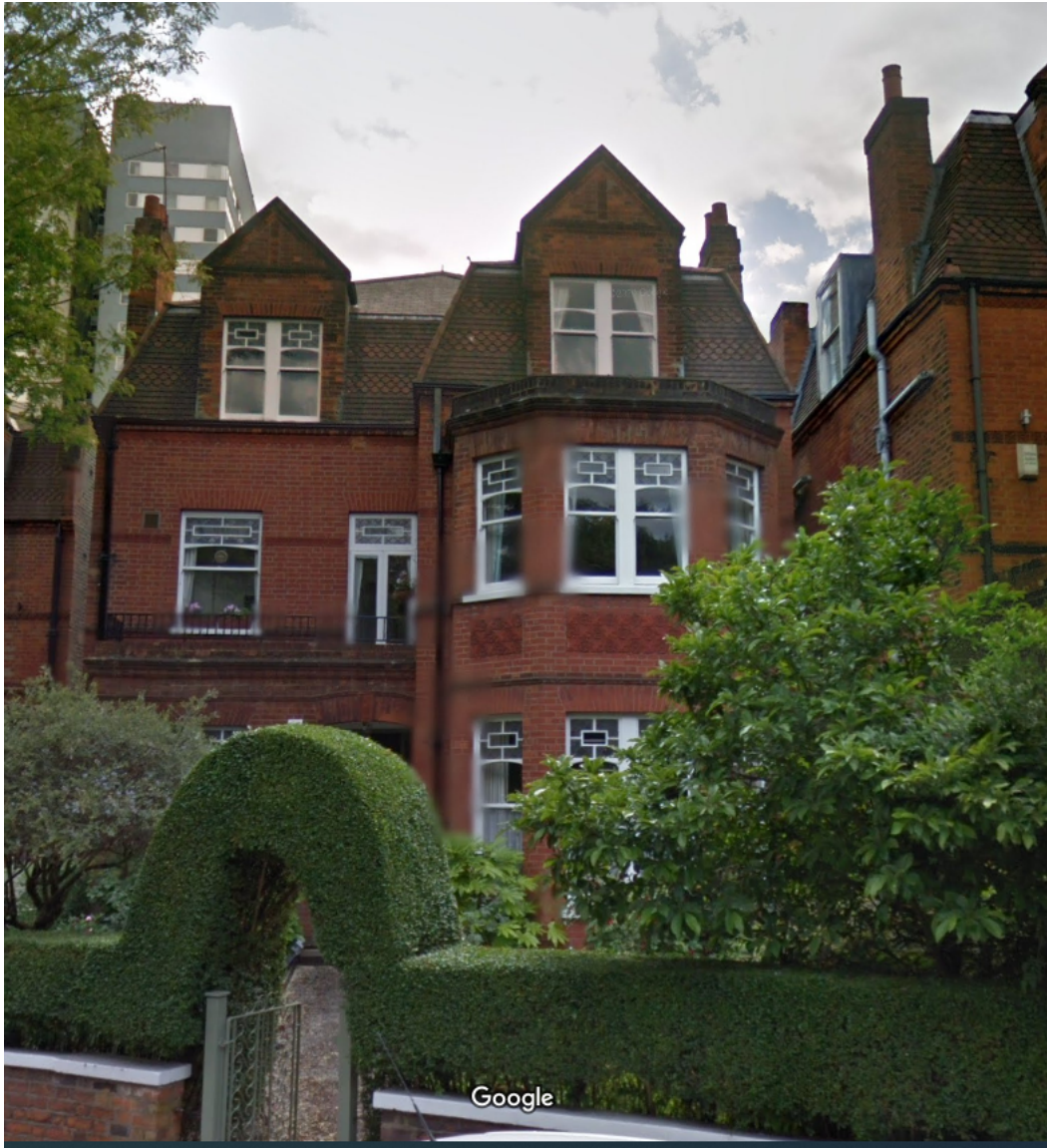
View of front elevation from the street
