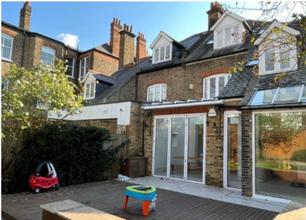
3. Photo of existing rear elevation and neighbouring rear extension
