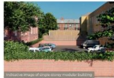
Indicative image of single-storey modular building
