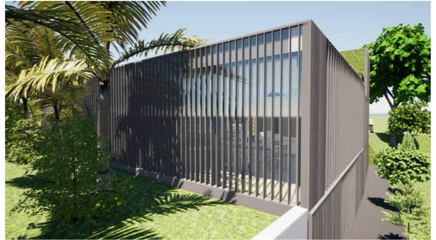
Corner South-East View
