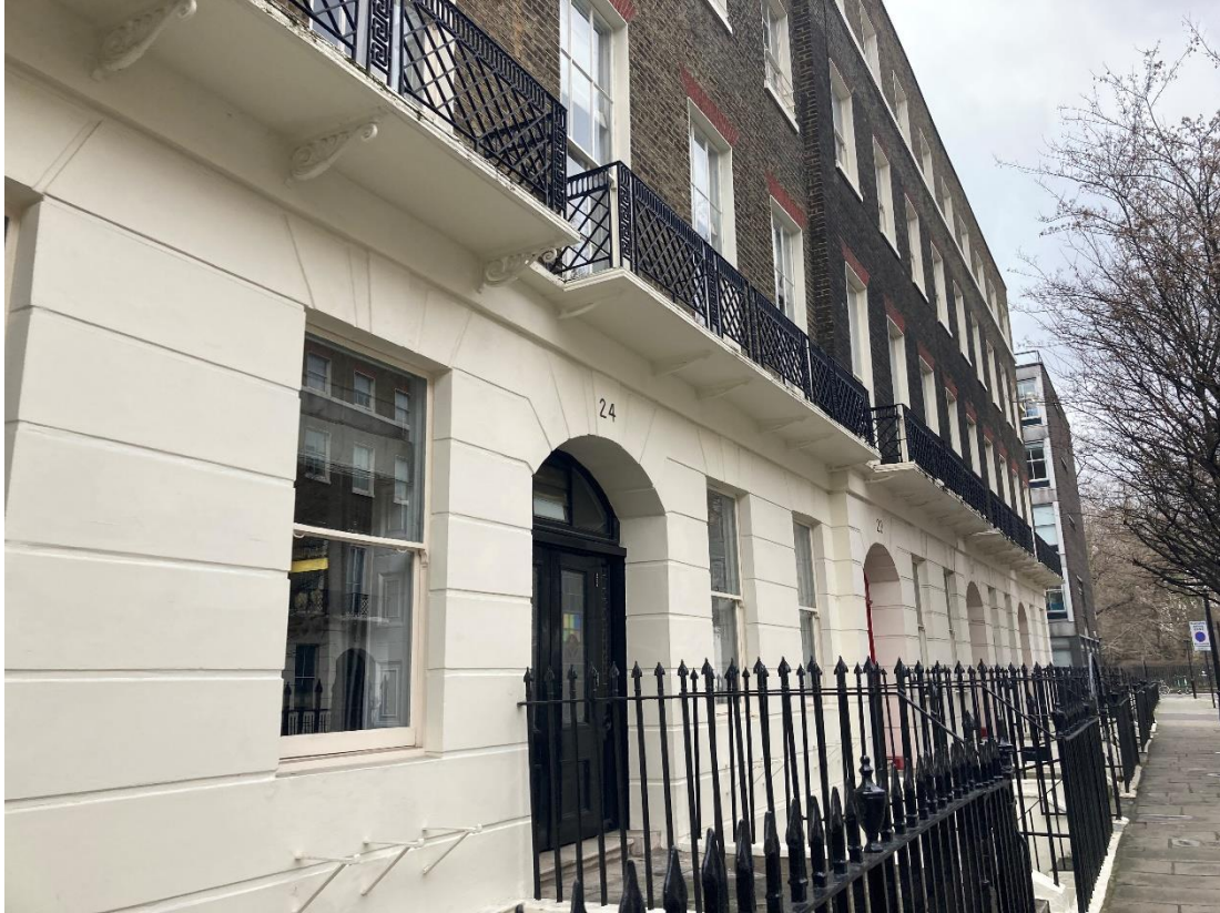
Figure 2 - 21-40 Bedford Place, showing the balconies at first floor.
