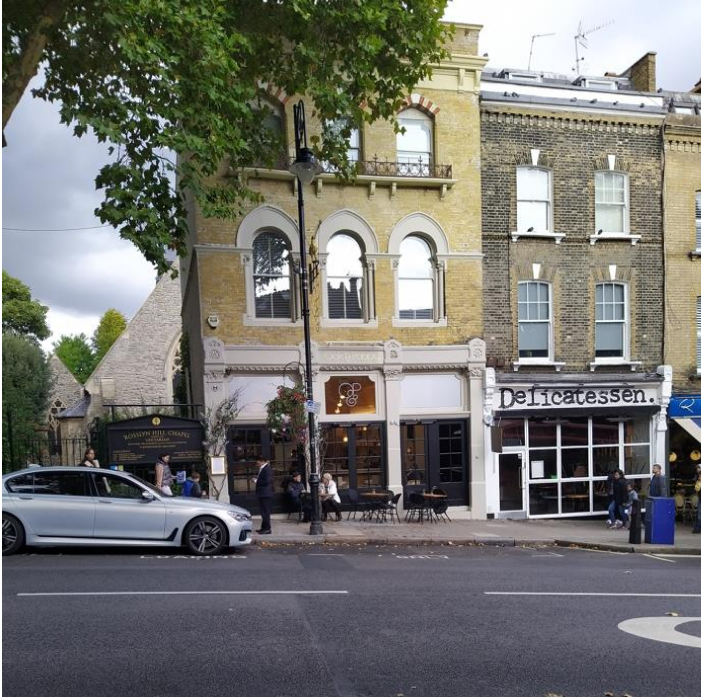
Figure 1: Existing shopfront at 48 Rosslyn Hill
