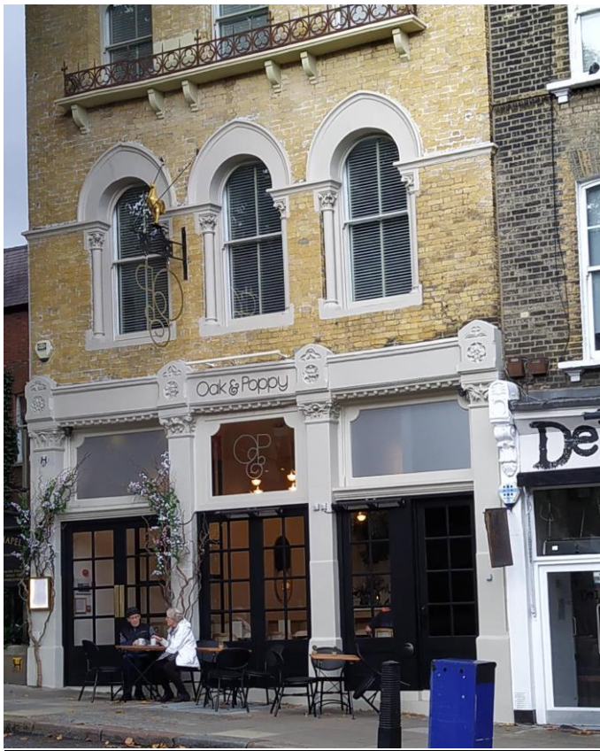
Figure 6: As built shopfront with heat lamps
