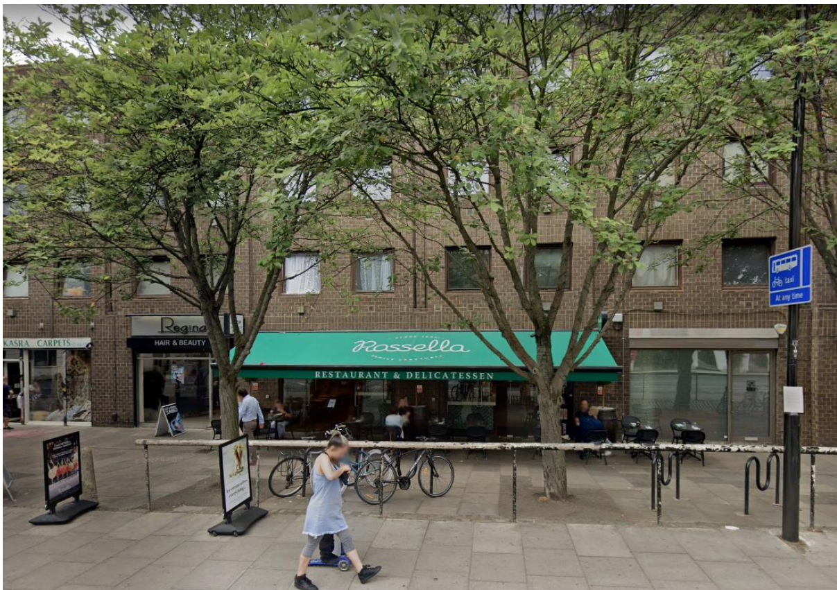
Photo 2 (above): Front elevation of Rossella restaurant from Highgate Road
