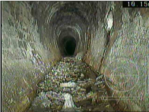
1404X_67ff0eed-1d31-49f8-8fce-9041d2d427ea_20201126_2 24005_535.jpg, 00:01:57, 10.15 m Settled deposits, other, 20% cross-sectional area loss, change, STONES.
