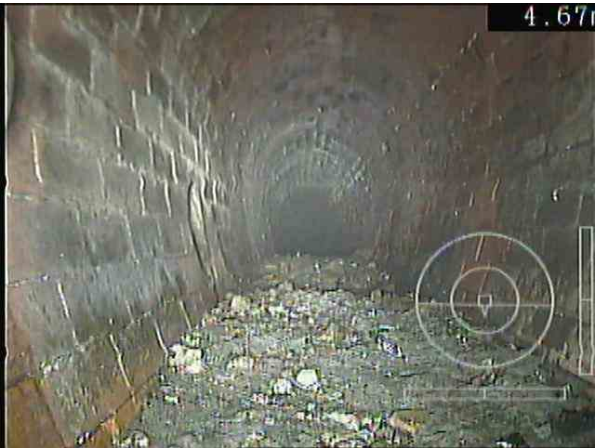
AX_039c8bfd-4d4b-45ac-80fa-ef92923d29bc_20201126_214340_704.jpg, 00:02:39, 4.67 m Settled deposits, other, 25% cross-sectional area loss, MISC DEBRIS.
