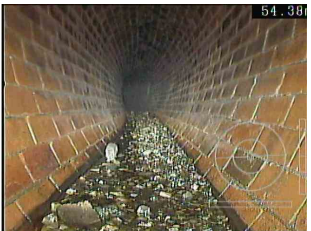
2410X_7e3257b2-c1f8-49bc-b568-69946098fc56_20201126_221344_246.jpg, 00:14:54, 54.38 m Settled deposits, other, 15% cross-sectional area loss, start, STONES/SILT
