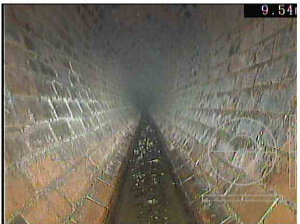
2410X_9ab88e92-d104-4df6-9a4f-2d35a0df584f_20201126_215846_440.jpg, 00:03:57, 9.54 m Settled deposits, other, 5% cross-sectional area loss, start, STONES.
