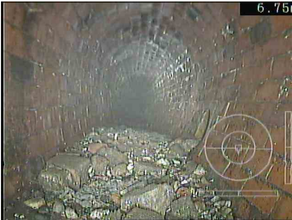
AX_d7a1fd96-2c30-402f-9ff9-2106f2f02221_20201126_214524_566.jpg, 00:03:56, 6.75 m Settled deposits, other, 30% cross-sectional area loss, BRICKS.
