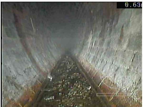
2410X_9b687413-1f07-4015-bba7-7a8cbe511628_20201126_215501_877.jpg, 00:00:03, 0.00 m Settled deposits, other, 10% cross-sectional area loss, start, SILT STONES.
