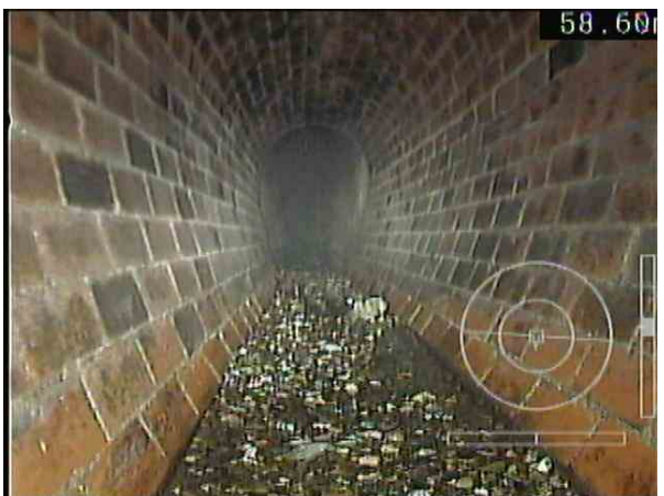
2410X_67116f1c-1756-4bb2-97ac-1c50c1808398_20201126_221459_733.jpg, 00:14:54, 54.38 m Settled deposits, other, 15% cross-sectional area loss, start, STONES/SILT
