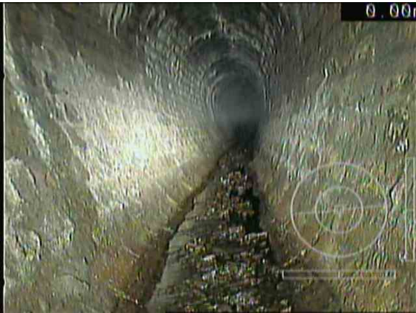
1404X_5a6a66f8-2045-4e38-bf52-cfa7817a955f_20201126_2 23747_361.jpg, 00:00:01, 0.00 m Settled deposits, other, 10% cross-sectional area loss, start, STONES.
