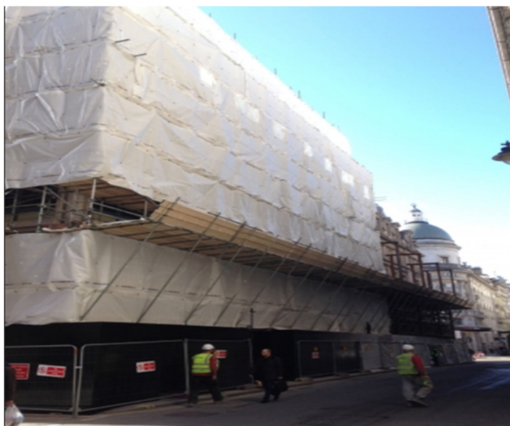
Figure 11: Typical hoarding with sheeting and fall arrest fans
