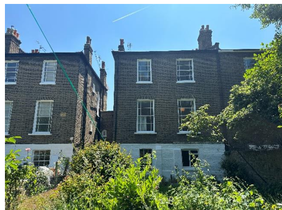
fig.3 view showing back of 100 Belsize Road
