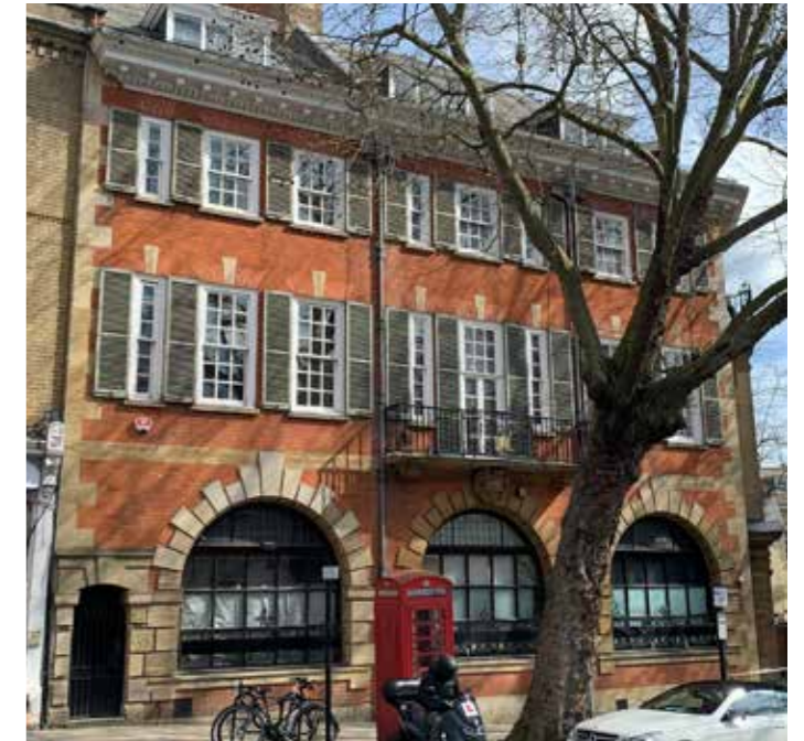
Figure 4.2 Principal south elevation of the building. Remains of window signage are visible at ground floor level.
