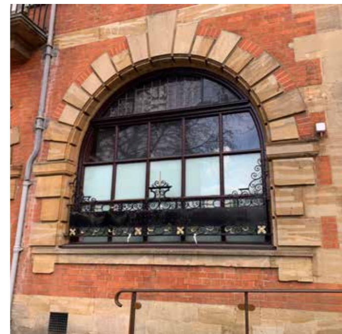
Figure 4.1 Example of a sign mounted to the railing of windows located at ground floor level. The boarding for the sign remains in-situ, however the lettering of the former 'Lloyd's Bank' sign has been removed.
