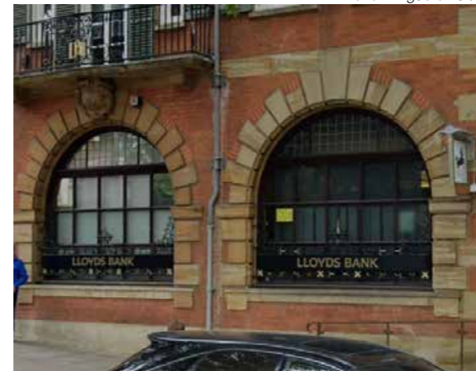
Figure 5.3 New signs affixed to the window sign boards. The signs are the same size and present a similar design to the former 'Lloyd's Bank' signs which were previously located here.
