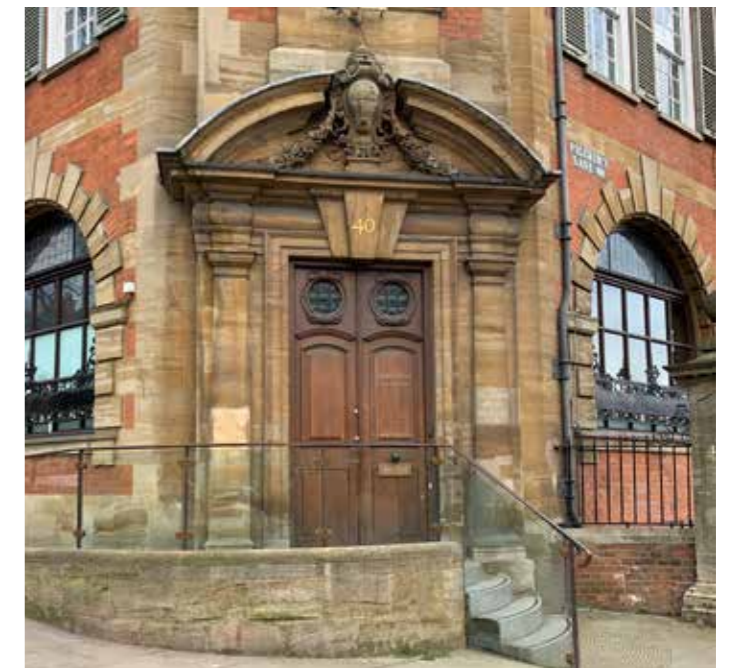
Figure 4.3 The stone doorcase with modern disabled ramp, installed in 2004 following Listed Building Consent. Stonework to the left of the arched pediment presents evidence of a former sign
