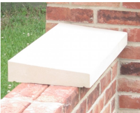
09. Stone - Copping for Parapet Wall
