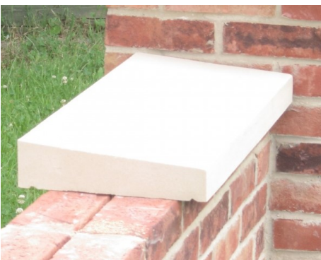
09. Stone - Copping for Parapet Wall
