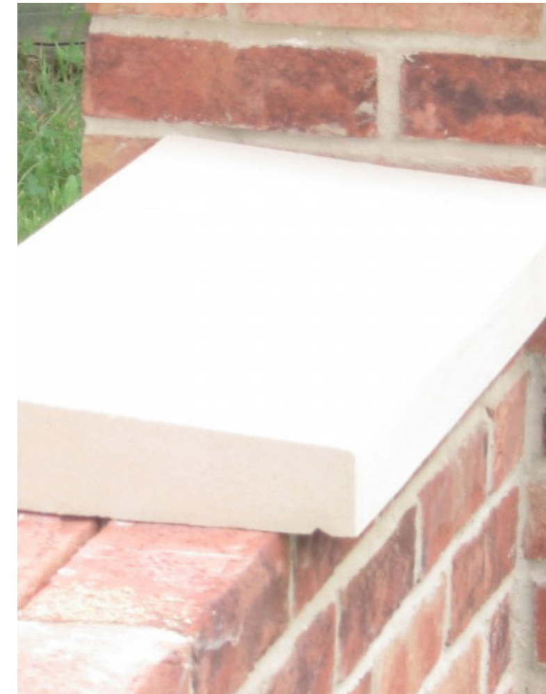
09- Coping of parapet Wall
