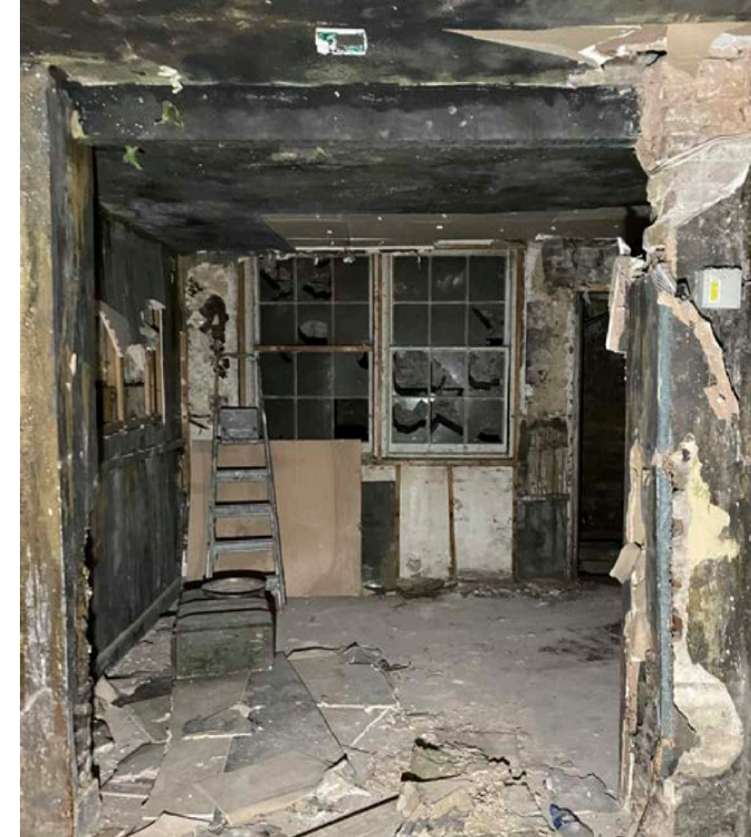
Modern joist supporting opening to front and back of basement. Boarded up fireplace possibly concealing range. Concrete screed.
