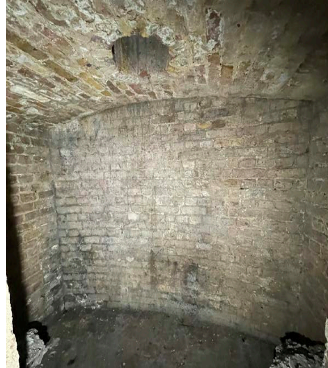
Front vaults and coal hole
