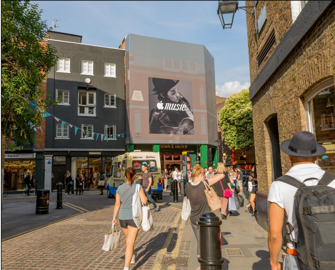
Fig 7: Example of the aesthetic benefit afforded by a scaffold shroud.
