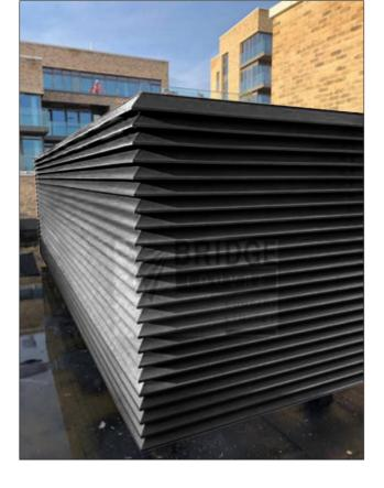
Proposed form of roof top louvred plant screen To be finished in RAL 7016 Anthracite Grey
