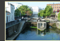
Hampstead Road Locks, 1819
