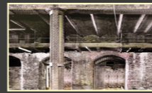
Interchange Basin ("Dead Dog Hole") view to Wine & Beer Vaults
