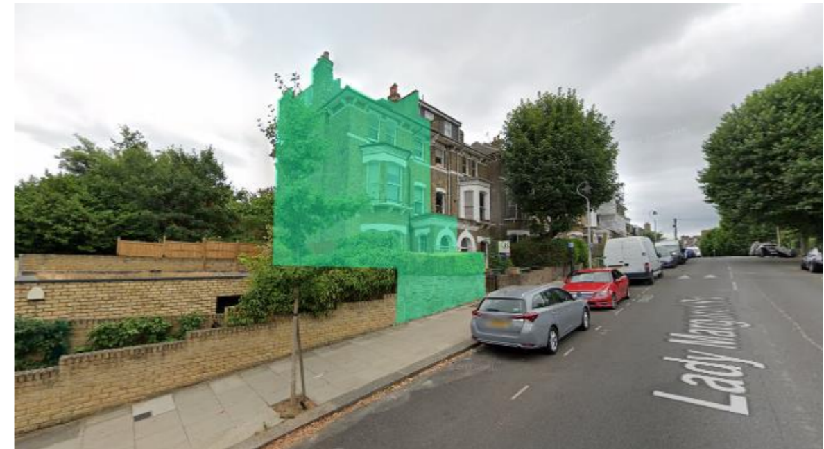
Figure 2 - Street view from Lady Margaret Road looking south-West with building highlighted.
