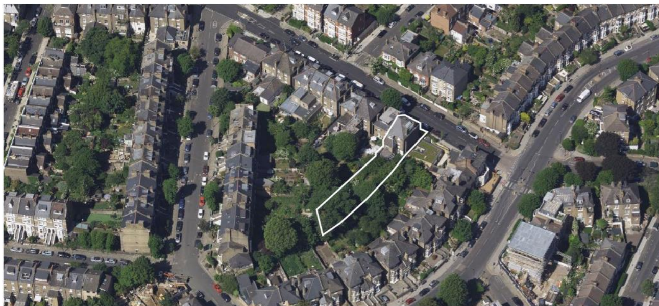
Figure 1- Site view showing the site highlighted (Novak Hiles Architects Planning Material)
