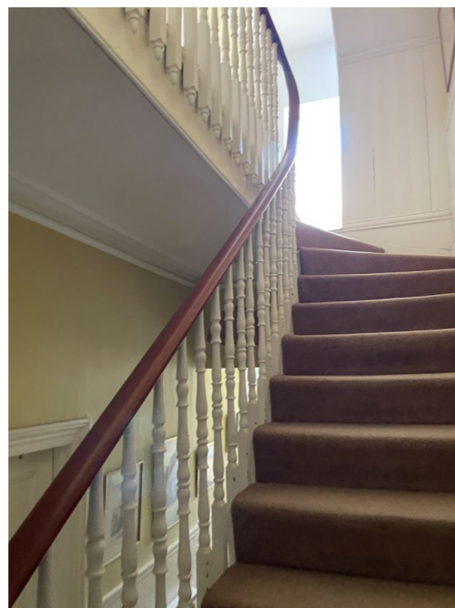
Original Stair Handrails
