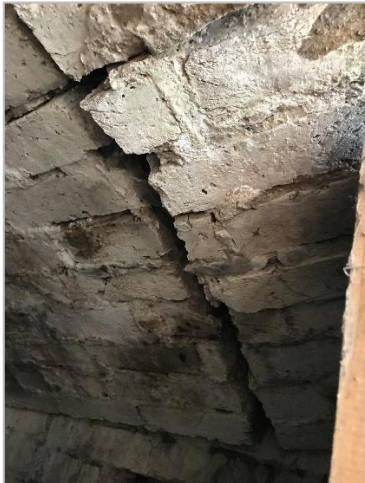
3. Separation of masonry within vault roof structure
