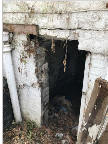
4. Current condition of degraded vault entrance
