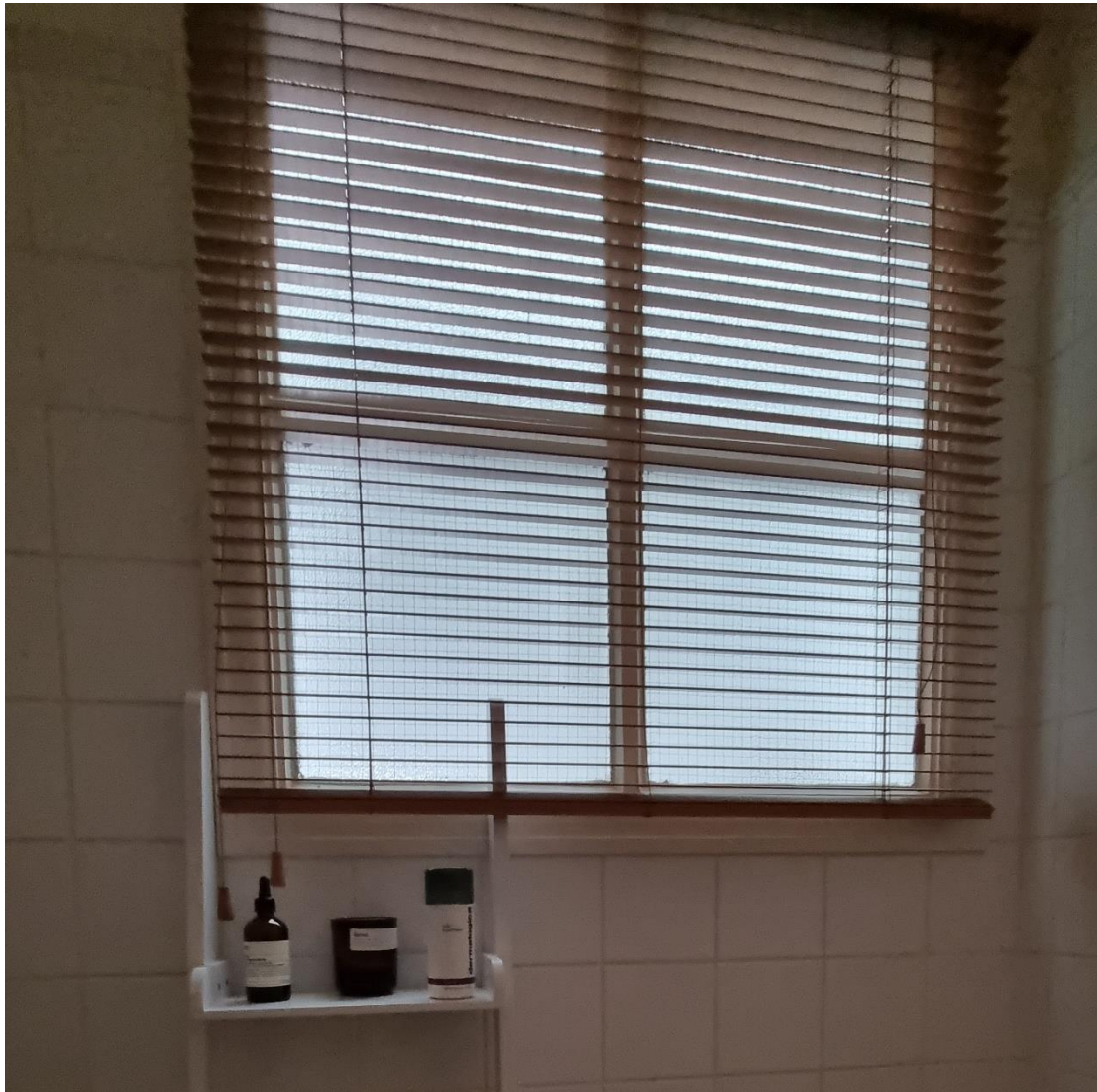
Fig.20: Bathroom window to internal lightwell.
