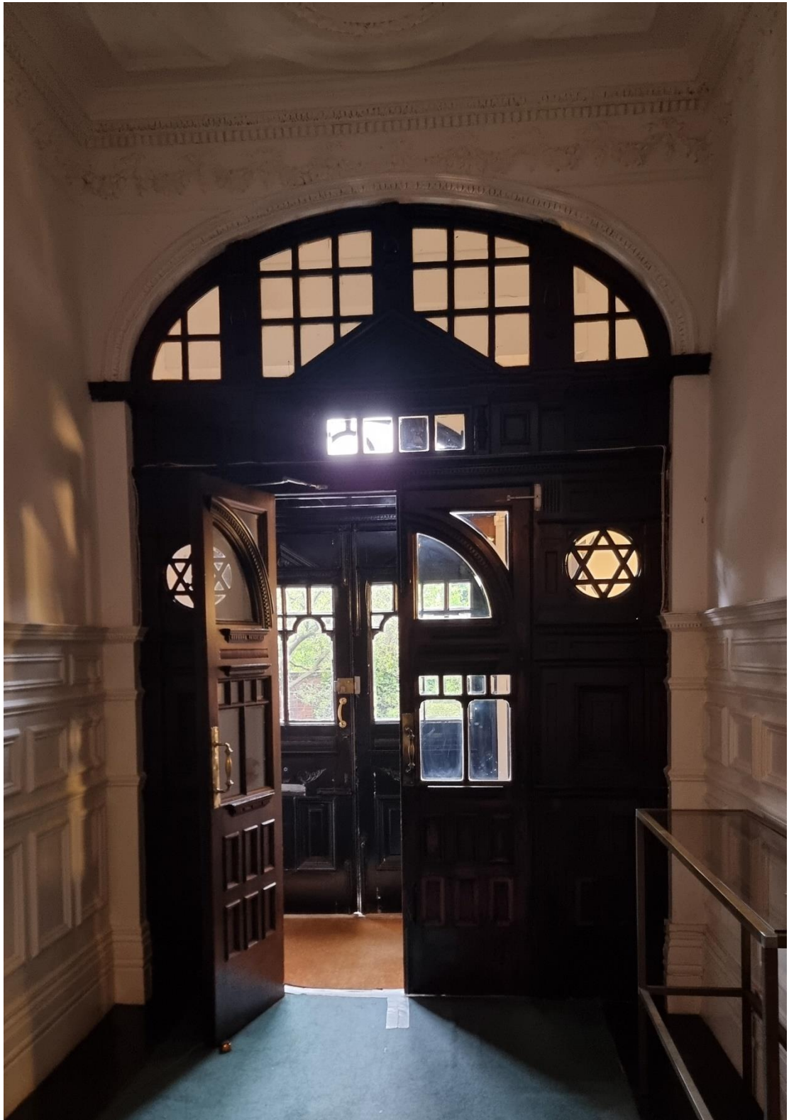
Fig.9: Internal view of shared main entrance door.
