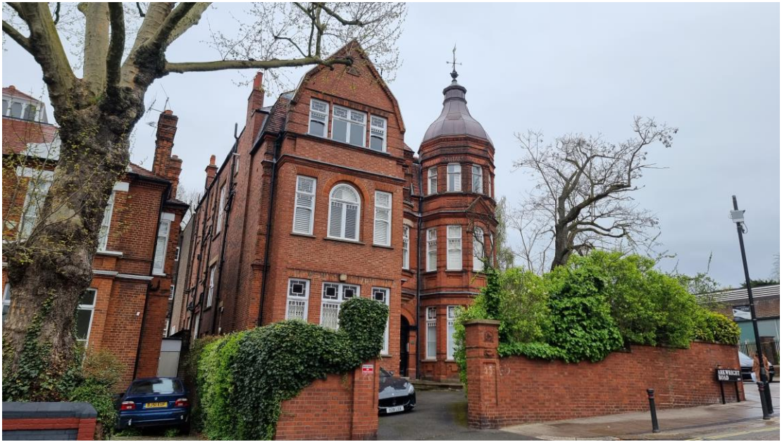
Fig.3: Access to southern side on Arkwright Road.
