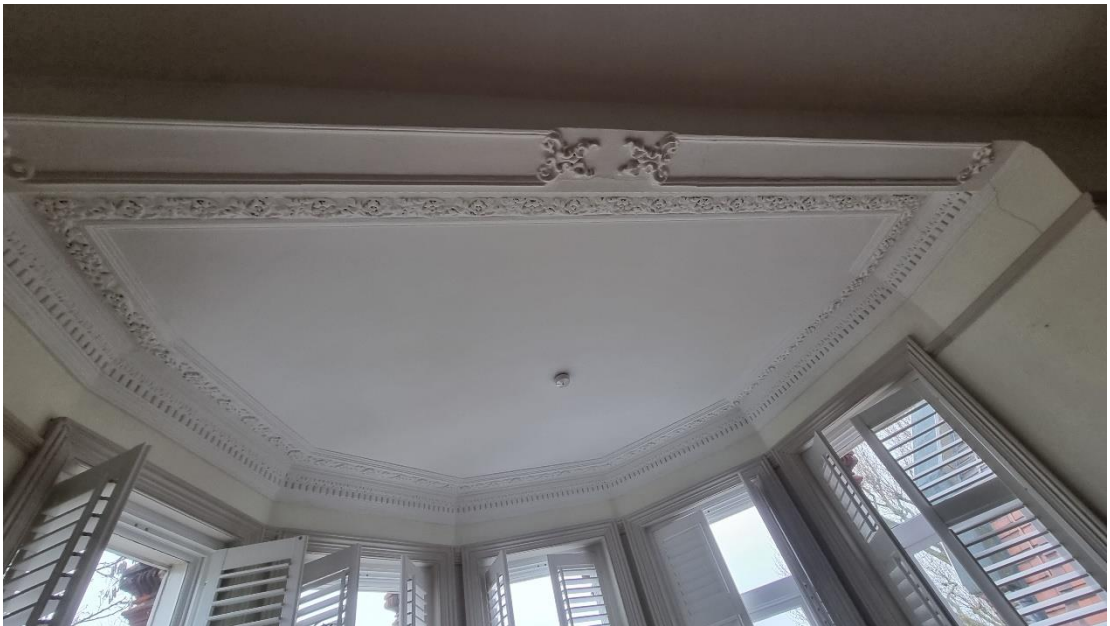
Fig.16: Ceiling detail of the turret in the living room.
