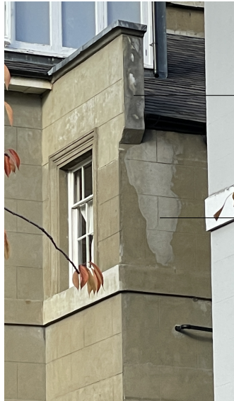
Photographs of local repairs to Roman cement, in lime plaster
