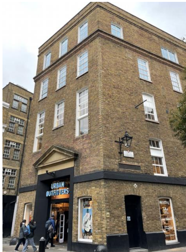
Figure 24 Front façade of the Seven Dials Warehouse
