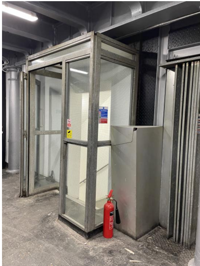
Figure 18 Entrance to staircase
