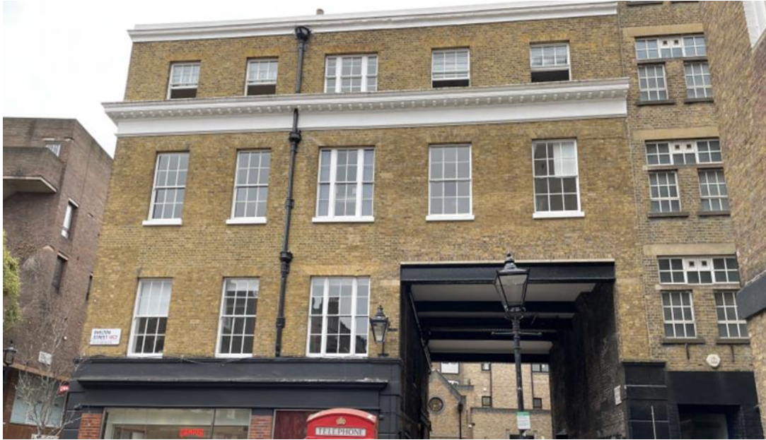
Figure 27 No. 34 Shelton Street and entrance to Brewer's Yard
