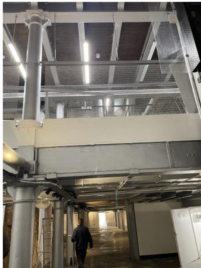
Figure 21 Double height ceiling area
