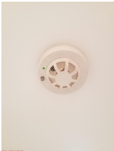
Entrance and Hallway, Ceiling, Smoke alarm tested and in working order
