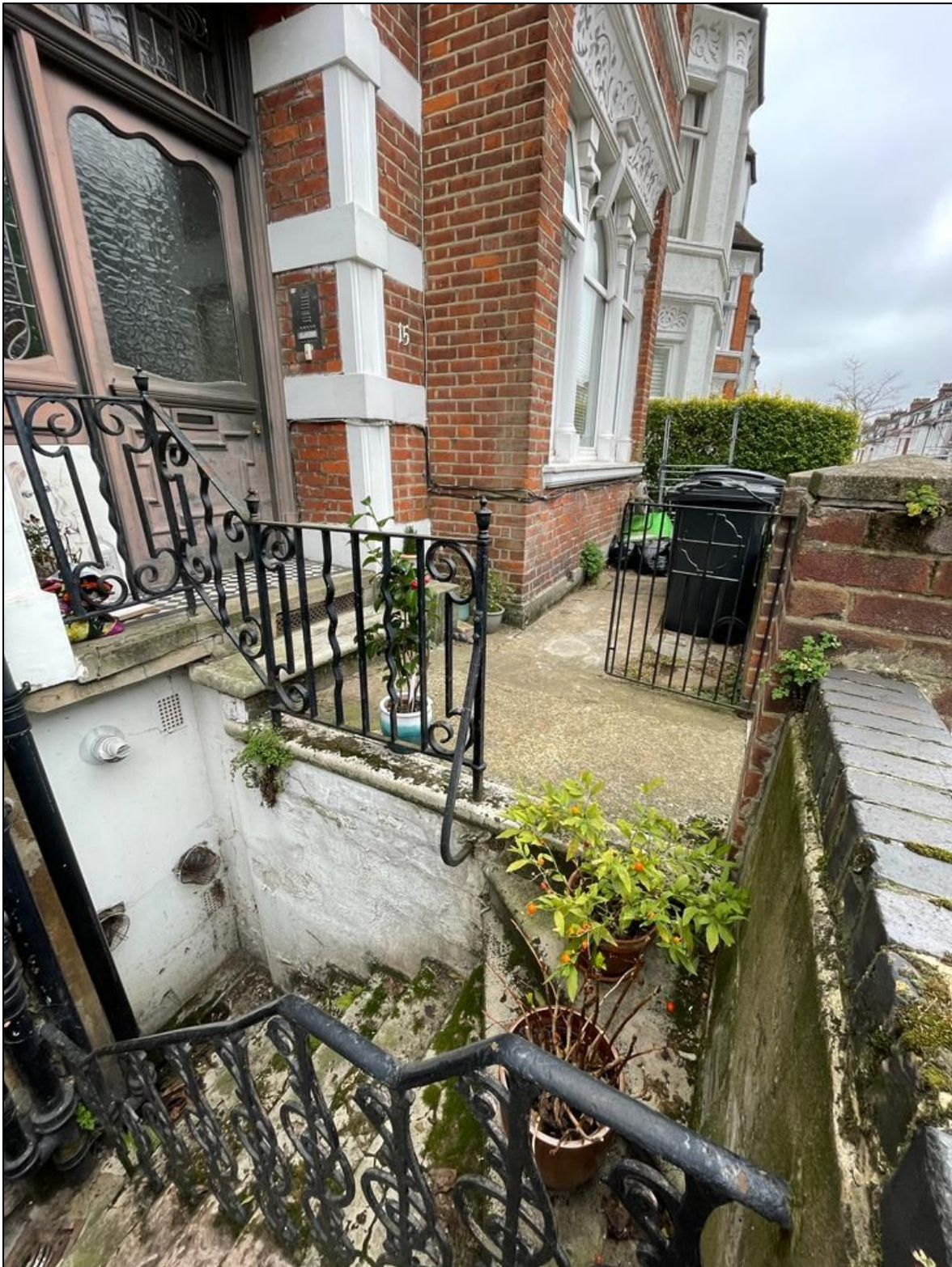
Photograph 2 – Taken of the front entrance, including the steps to the basement area.
