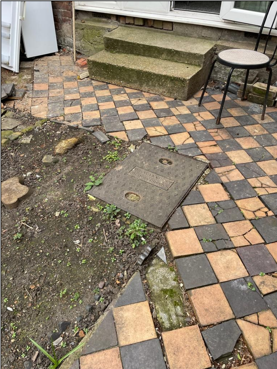
Photograph 5 – Photo taken of the manhole cover on site.
