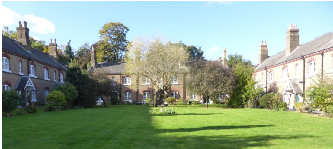
Fig. 24 overall view towards the West range
