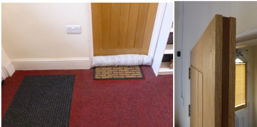
Figs. 25,26 Internal view showing new skirting and floor coverings with new FD 30 fire door
