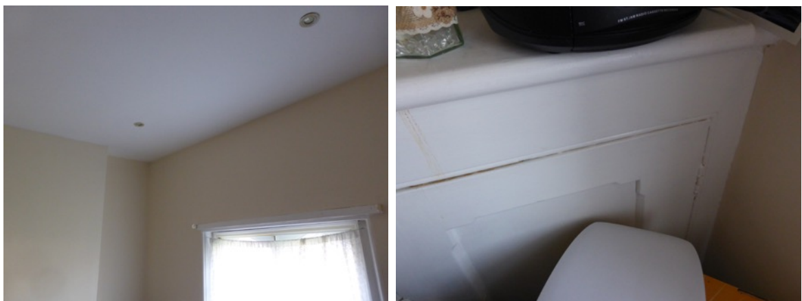
Figs. 28,29 existing plasterboard ceilings within the dwellings, the retained 'small timber cupboard
