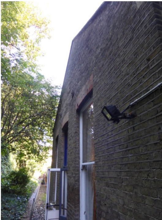
Fig. 21 West gable elevation to the Hall
