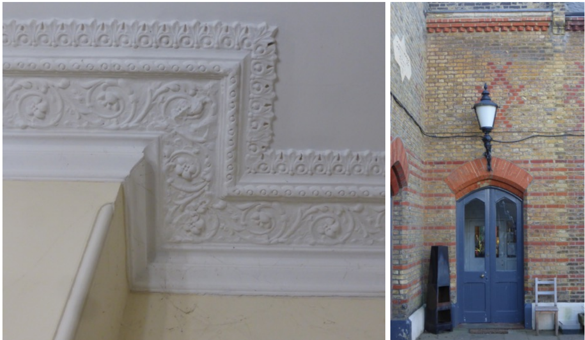
Figs. 12,13 Hall cornice, Hall courtyard entrance door
