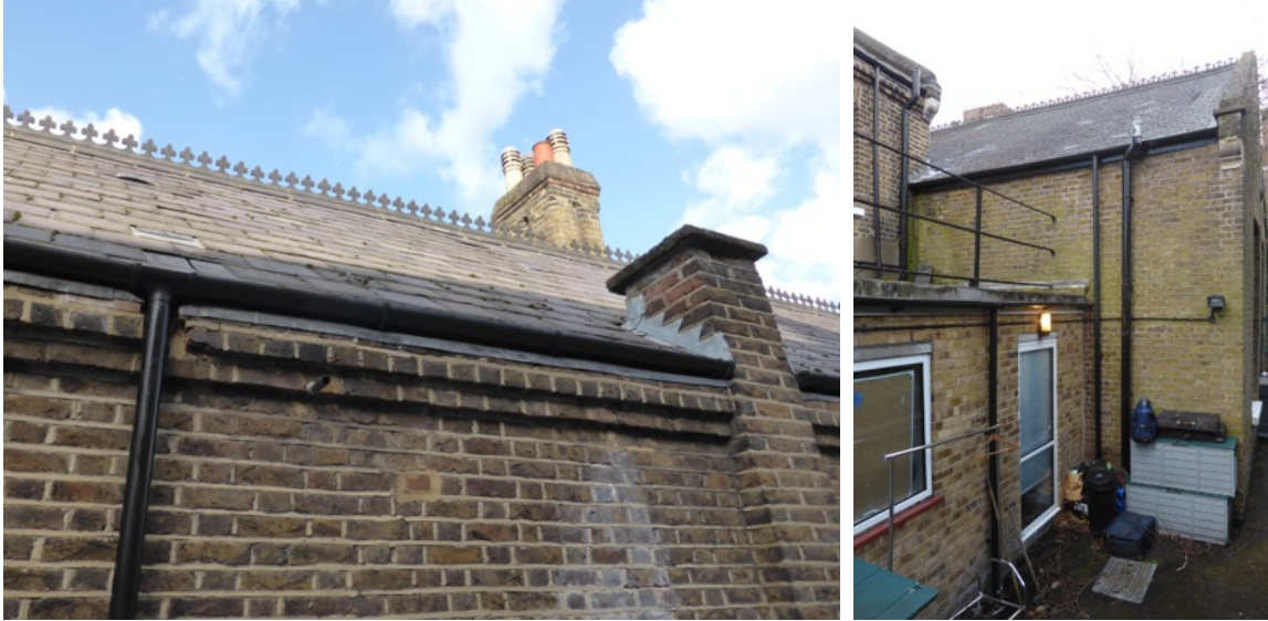
Figs. 19,20 South and North elevations showing plain stock brick and PVC-u drainage
