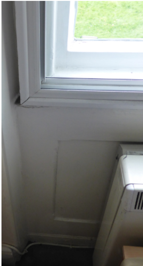
Fig. 30 existing timber panel below the courtyard windows
