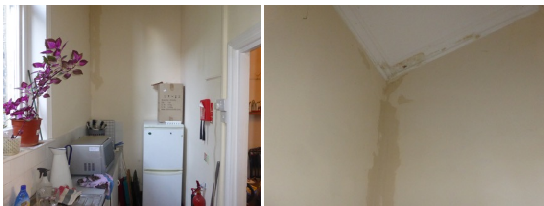
Figs. 17,18 Existing kitchen (West/Hall wall) and existing kitchen cornice.
