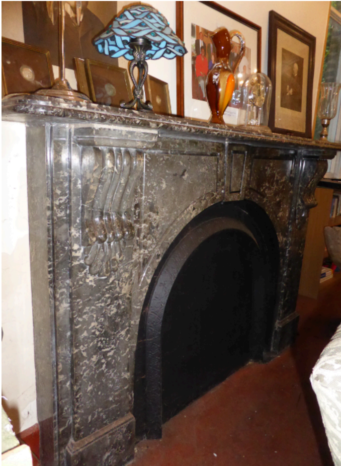
Fig. 14 Original fire surround with screed/linoleum replacing the missing hearthstone
