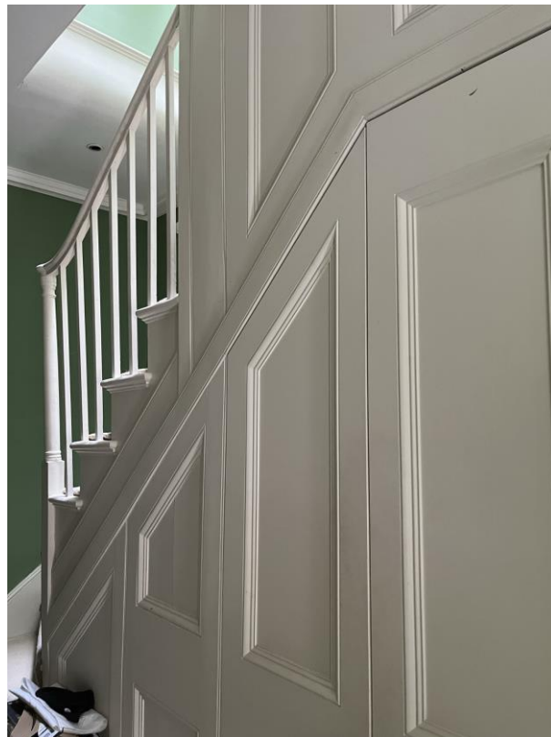
Photograph 36: Staircase with panelling to upper floors
