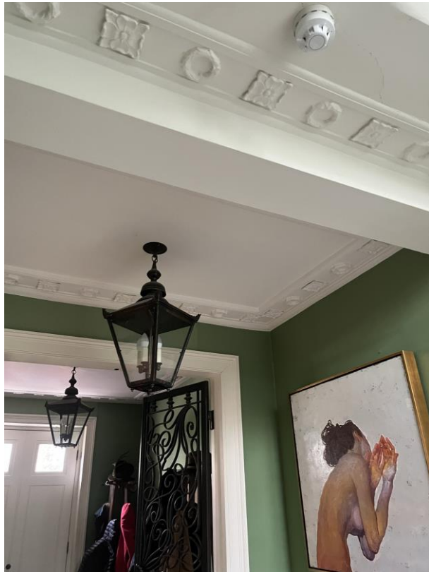
Photograph 14: Ground floor hall way with cornice detailing
