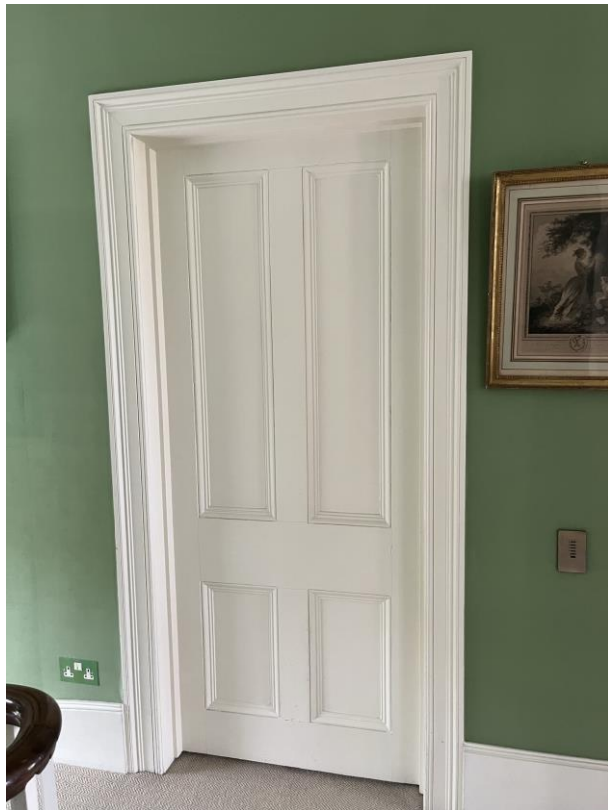
Photograph 27: Retained door to first floor
