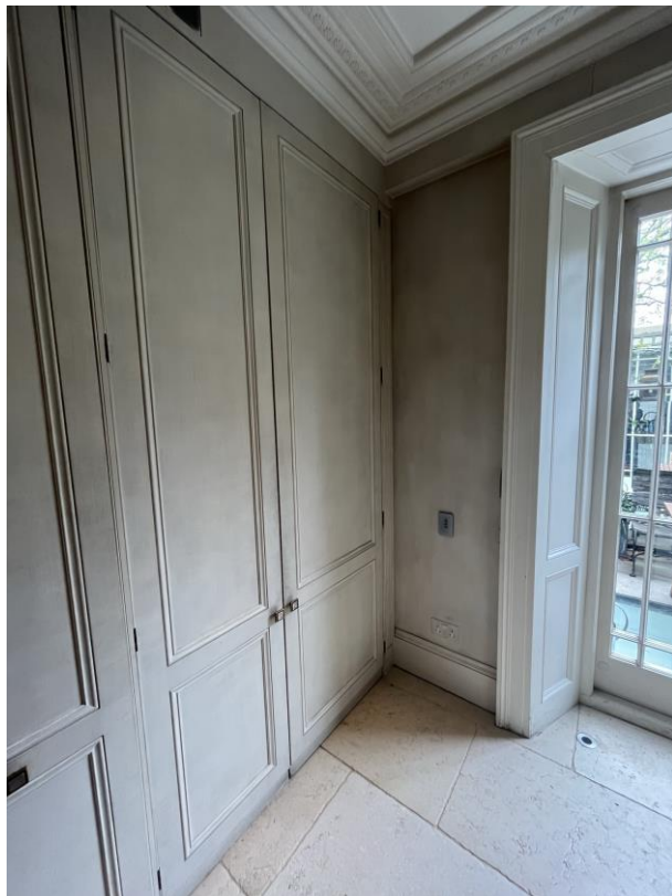
Photograph 8: Ground floor kitchen joinery door to pantry (closed)
