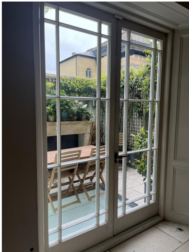
Photograph 6: Ground floor kitchen doors
