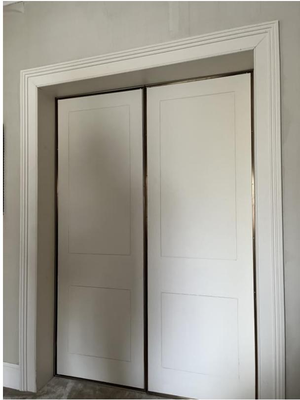
Photograph 33: Opening between front and rear rooms at second floor level
