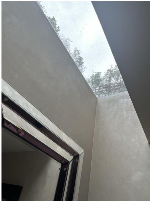
Photograph 10: Rooflight in ground floor WC
