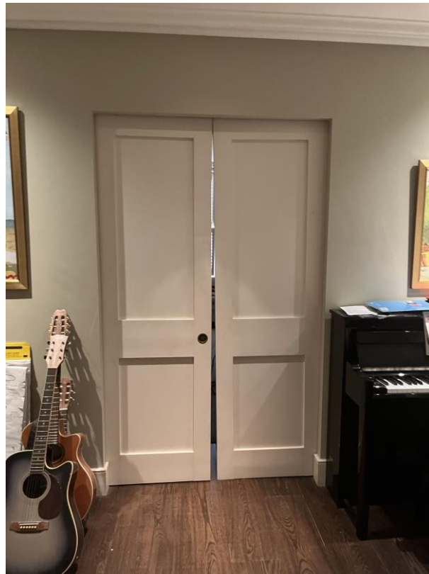
Photograph 20: Sliding door opening with new 'pockets' built on rear room side
