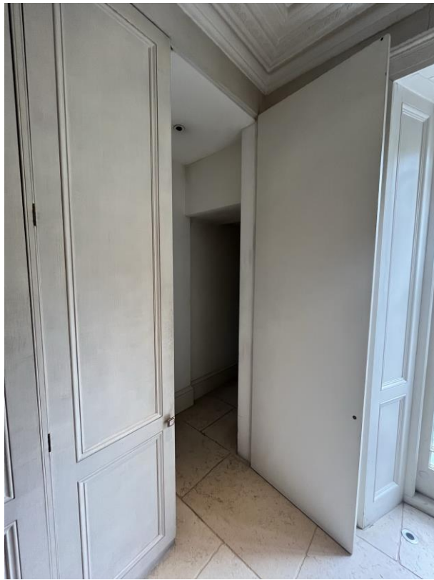
Photograph 7: Ground floor kitchen joinery door to pantry (open)
