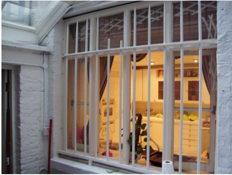
Photograph 3: Basement rooflight and window which was approved to be an opening
