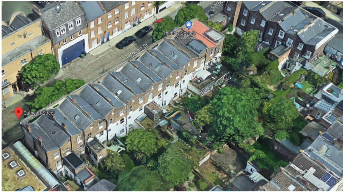
Aerial view of 1-9 Cathcart Street with No.5 at the centre
