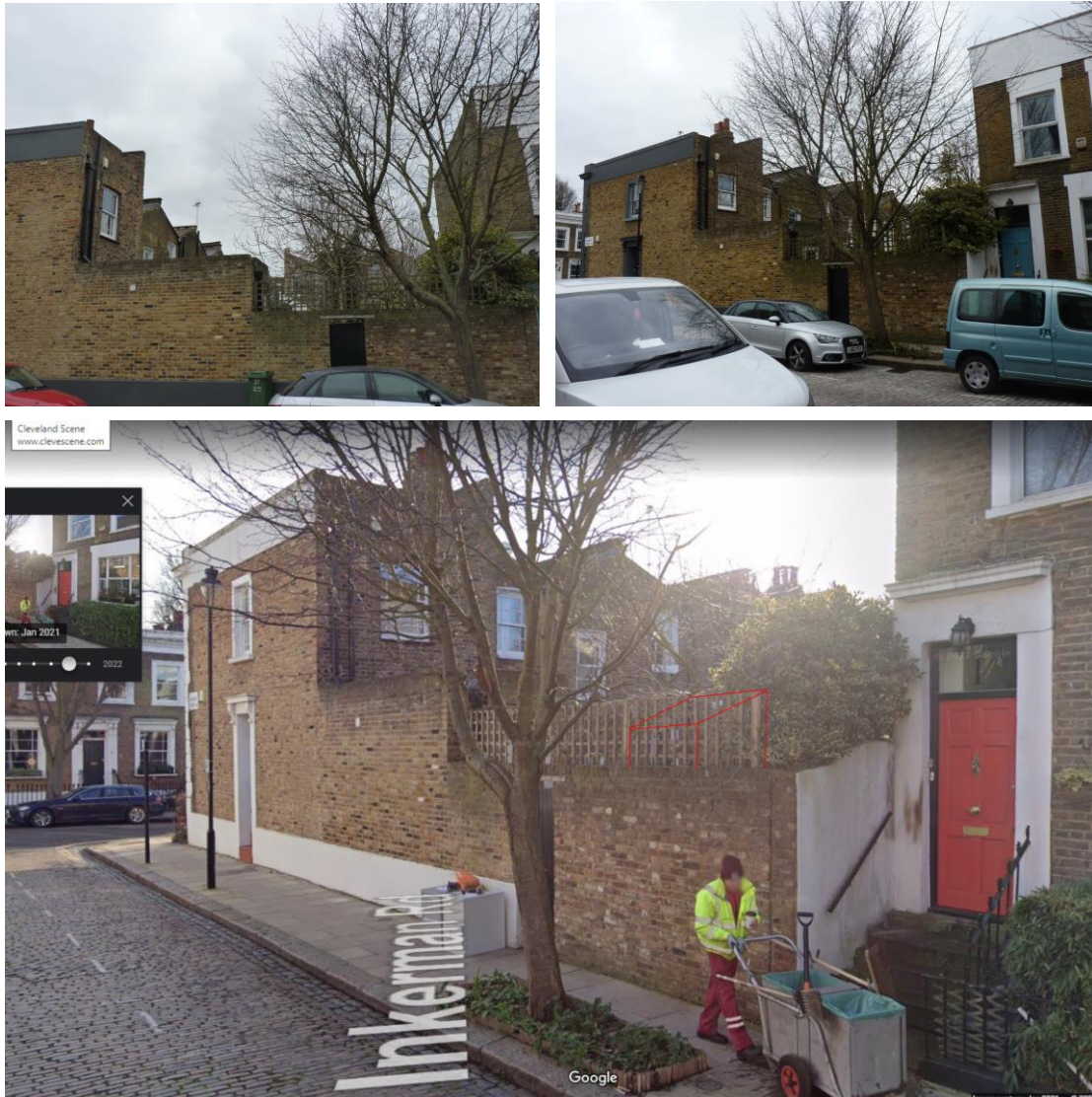
Views toward rear of Inkerman terrace from Cathcart St including graphic supplied to Officer
