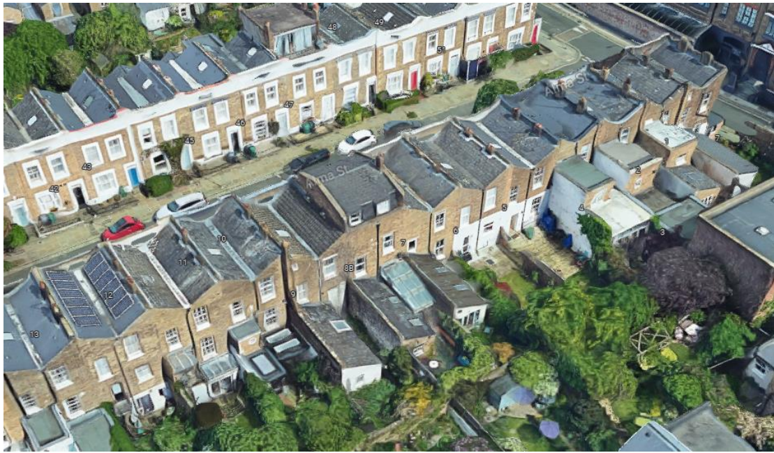
Aerial view to rear of No. 's 1-9 Alma Street
