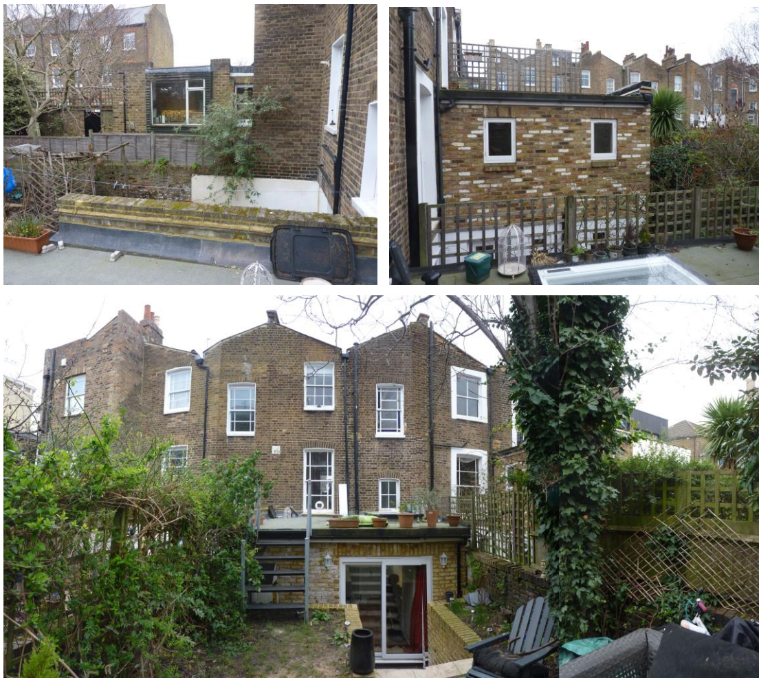
View to rear of terrace and of existing outriggers to No.'s 37 & 40
