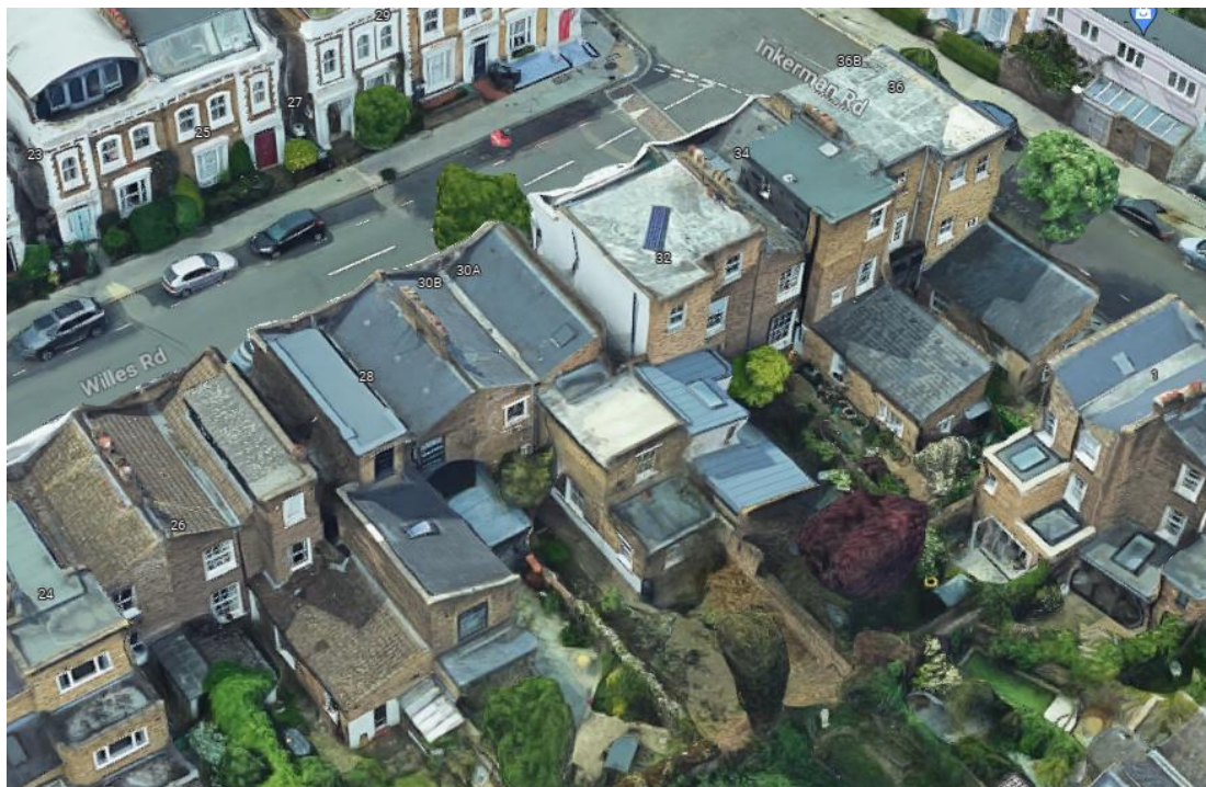
Aerial view to rear of No.'s 26-36 Willes Road
