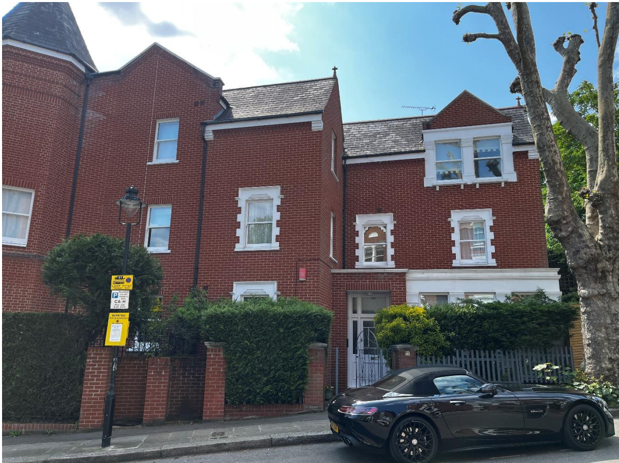
Figure 1: Photograph of the front elevation of 2B Tanza Road
