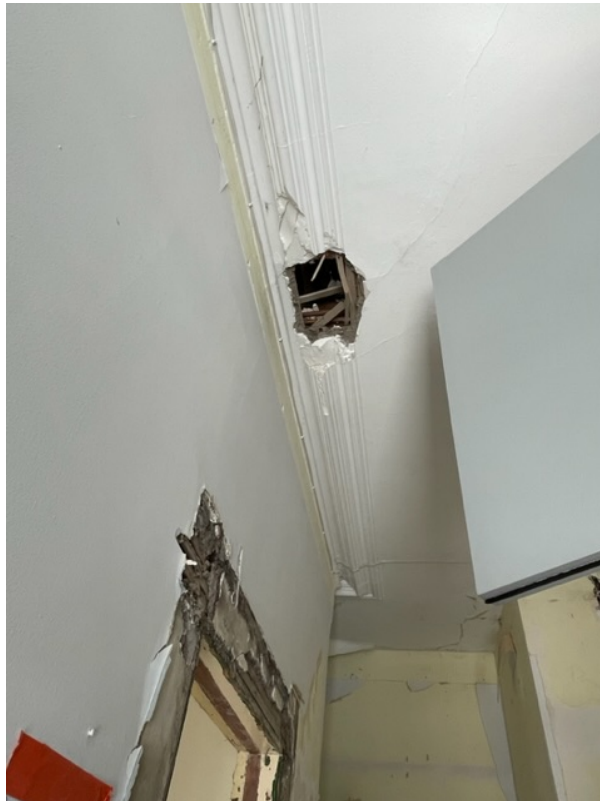
Evidence of lath and plaster walls/ceilings
