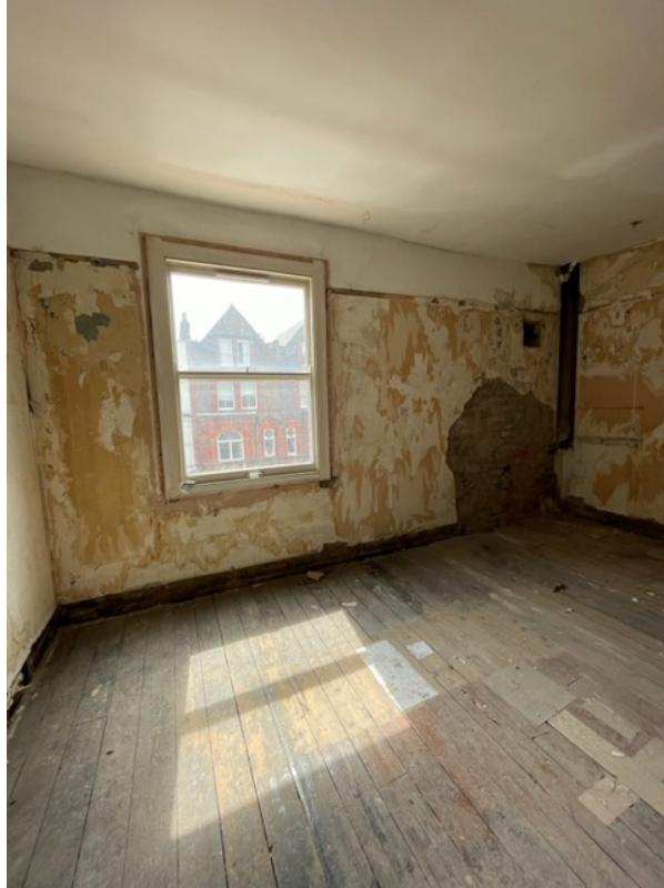
Example of removed plaster in small areas to expose brickwork
