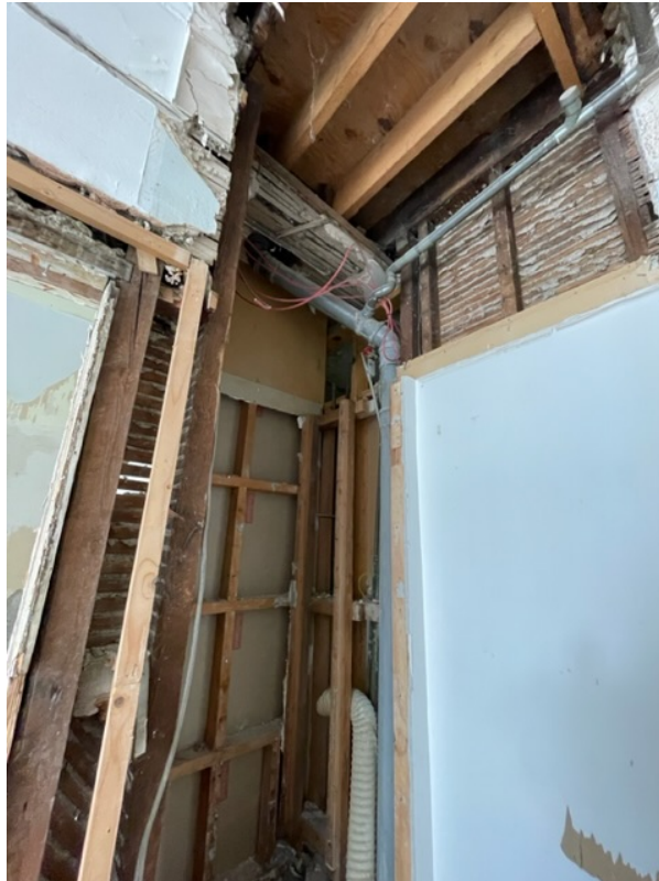
UGF flat separating wall to communal area stripped back
