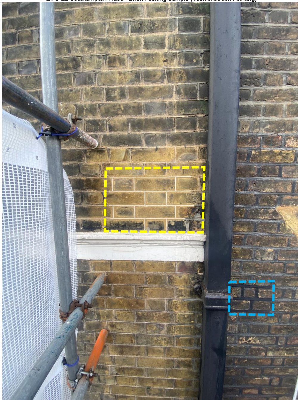
21 &amp; 22 Southampton Place - Brick Pointing Sample (Tuck &amp; Struck Pointing)
