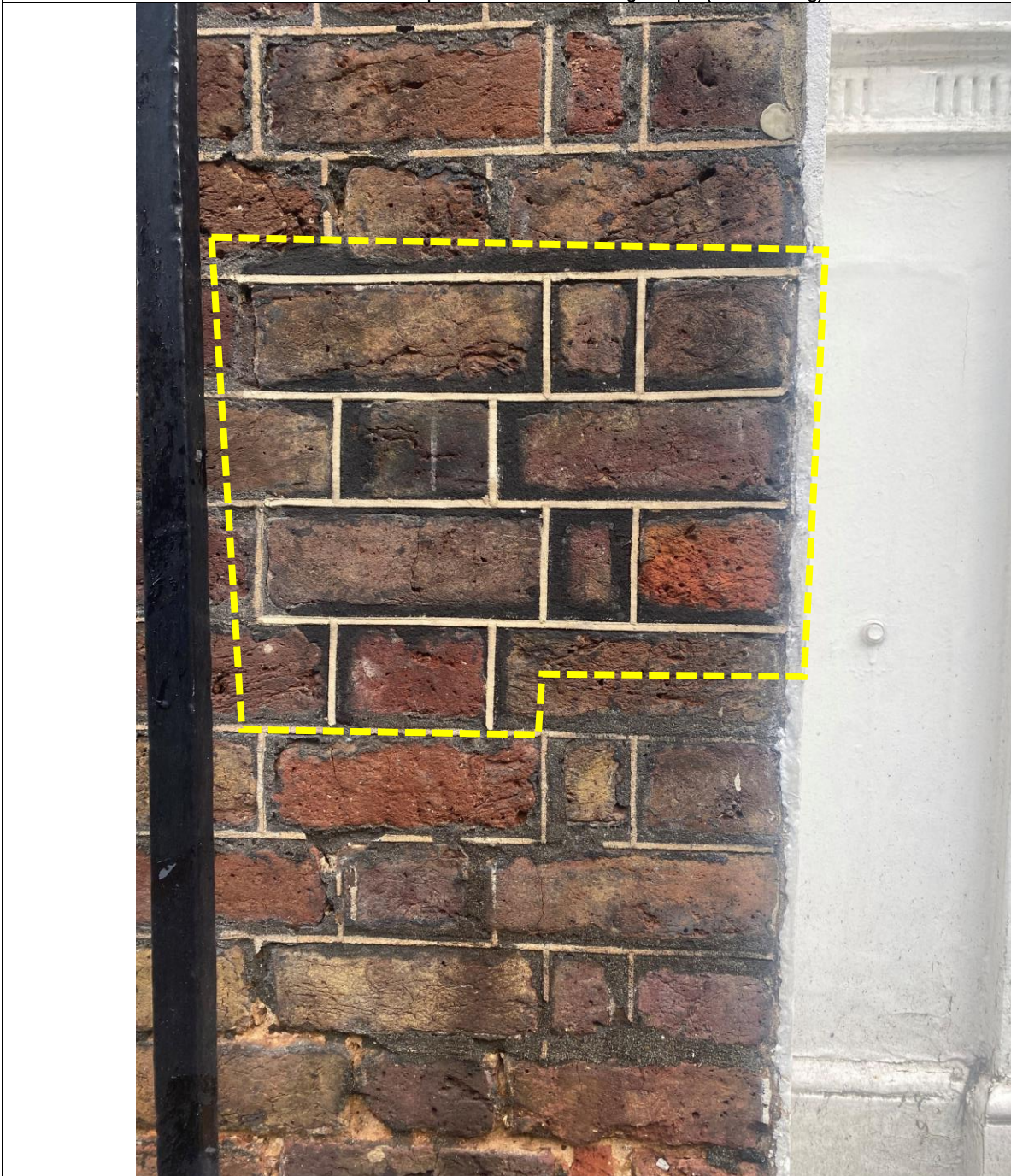
18 Southampton Place – Brick Pointing Sample (Tuck Pointing)
