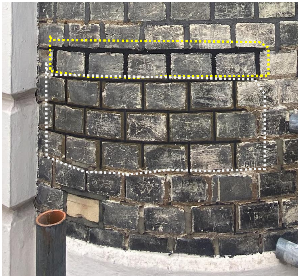
46 Bloomsbury Square - Brick Pointing Sample (Tuck Pointing)
