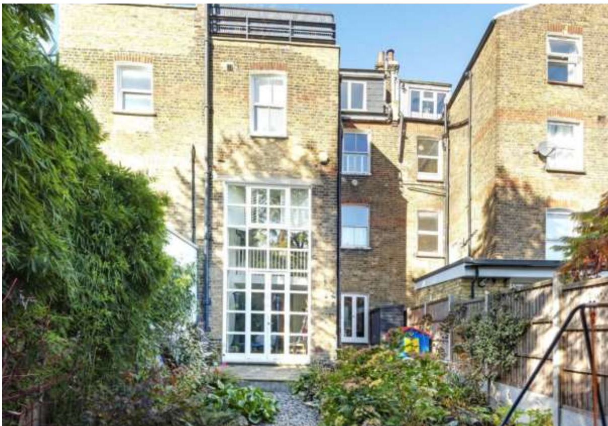
Roof terrace at no. 78 Hillfield Road
