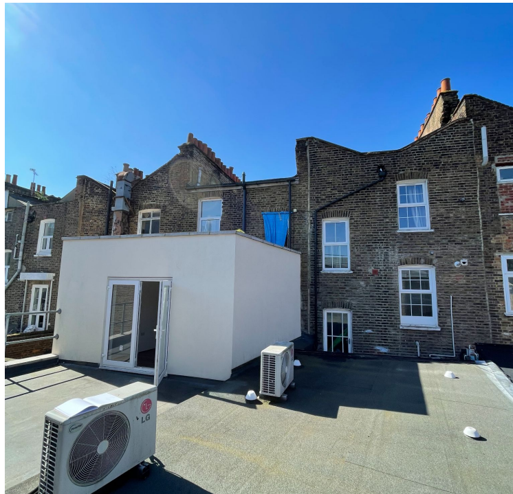
Image 1 - Single Storey Rear Extension at 240 Camden High Street
