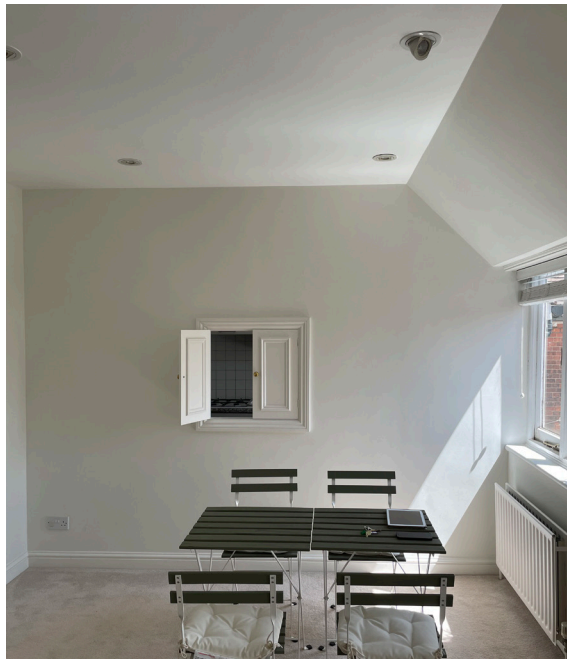
Flat 3. The partition dividing kitchen and main living space terminates within the window. The removal of the partition would bring the window/interior layout to its original configuration.
