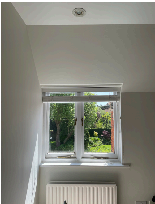
Flat 3, window W-G2. The partition dividing kitchen and main living space terminates within the window.
