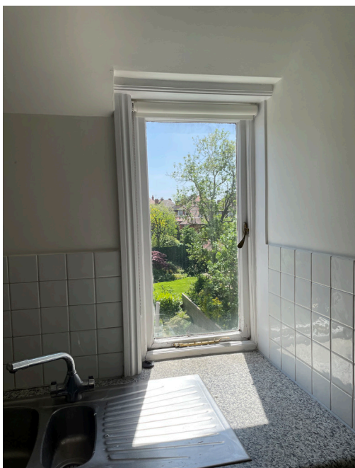
Flat 3, window W-G3. The partition dividing kitchen and main living space terminates within the window.
