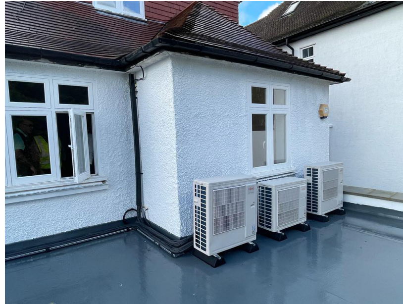
Air conditioning units, before installation of the acoustic enclosure
