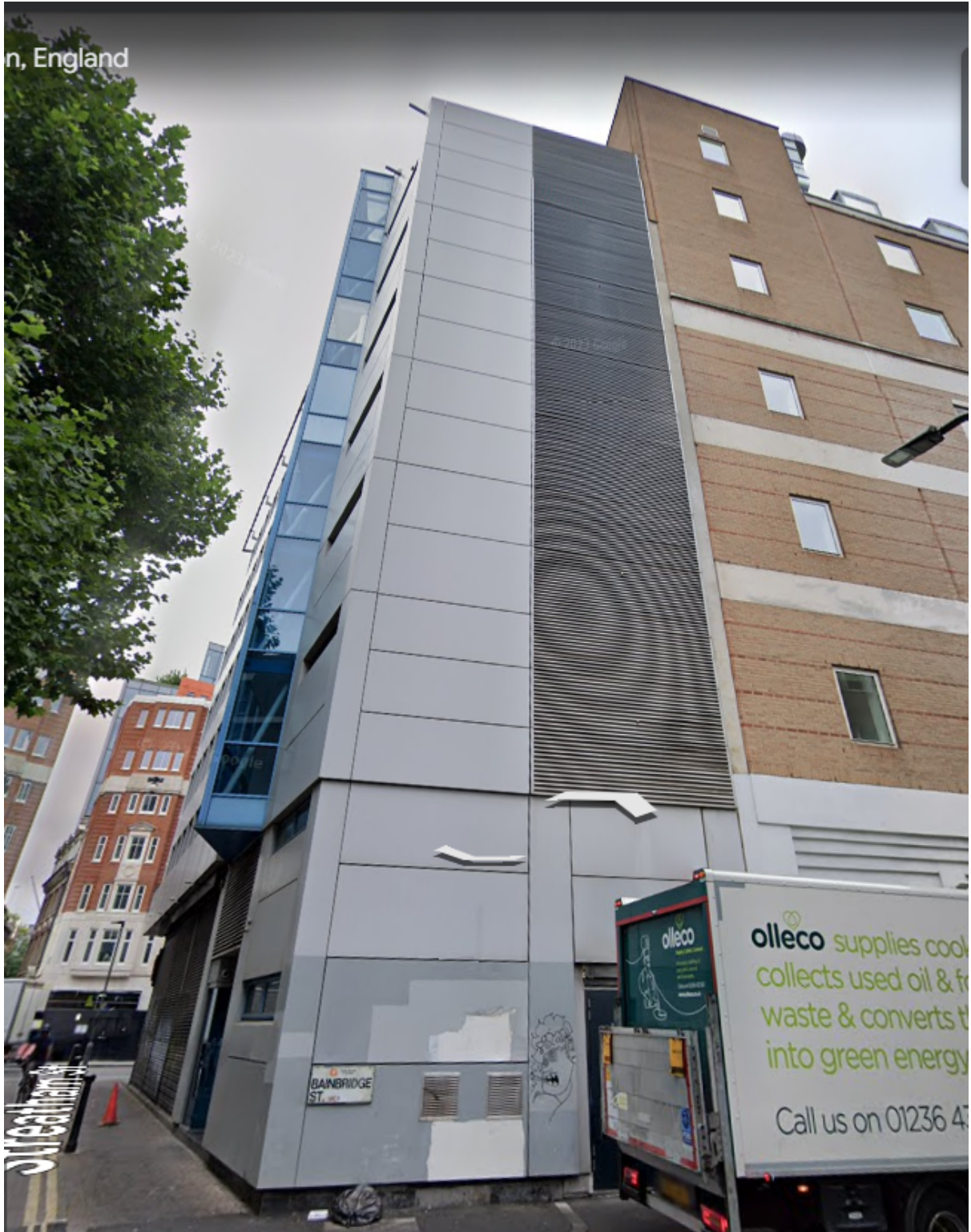
3. Photo of existing Bainbridge Street Elevation
