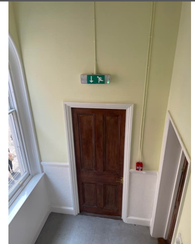
17.17.3 Door next to Flat A
