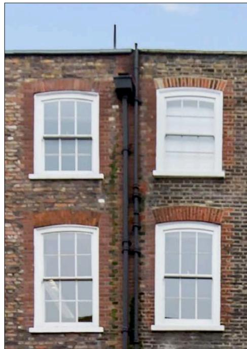
Photograph of the existing shared hopper (elevation view)
