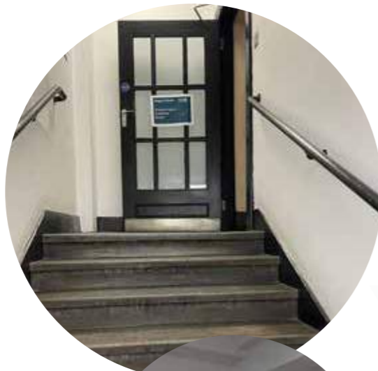
Uninspiring stairwell and low bulk head / ceiling.
