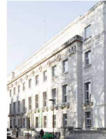
The Keppel St façade with regular openings
