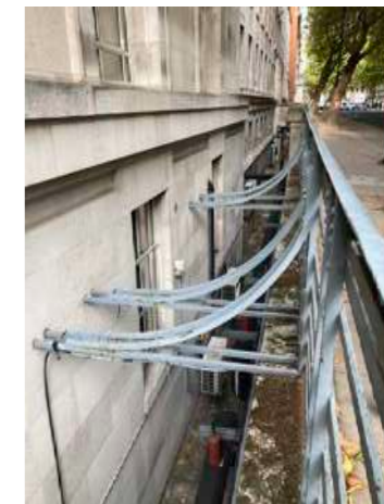
Metal brackets fixing railings to stone façade
