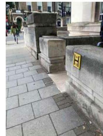
The stone parapet wall interrupted to provide access to the ramp
