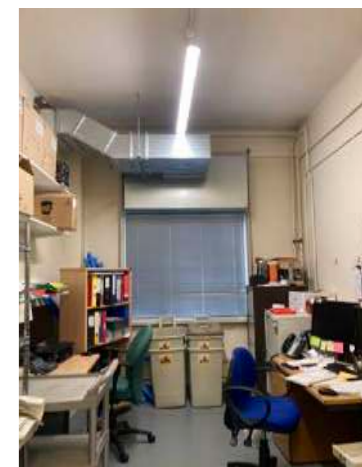
Storage room/ staff room
