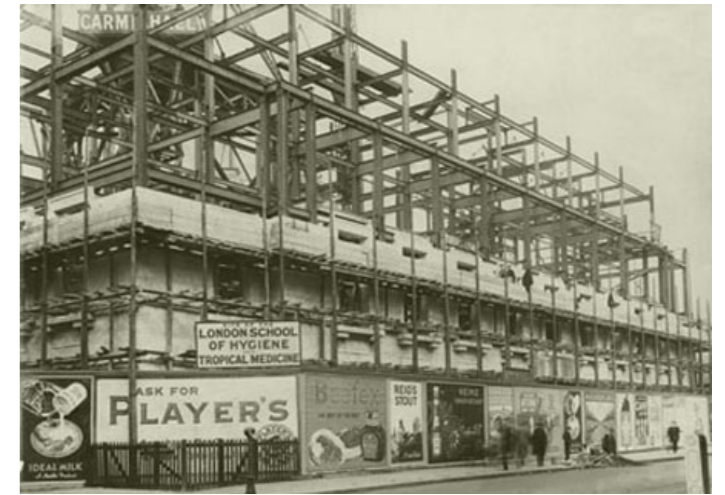
Steelwork under construction, 1926
