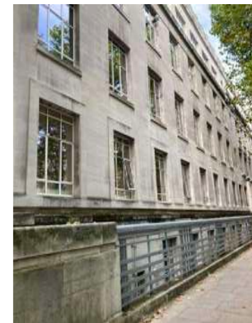
Metal railings on Gower St
