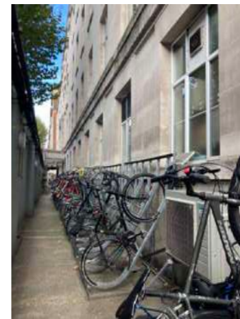
The moat cluttered with bicycles
