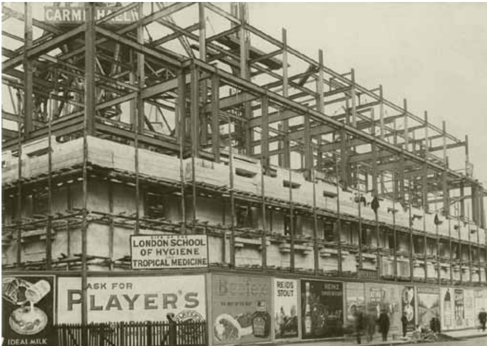
Fig 28. Steelwork under construction, 1926
