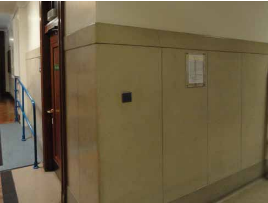
Fig. G13 terrazzo wall finish in corridor G04a
