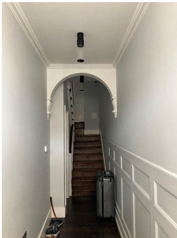
Figure 23: Remaining Entrance Hallway Dado Panelling, with Approved Blocking Up of Ground Floor Front Rooms Doorway
