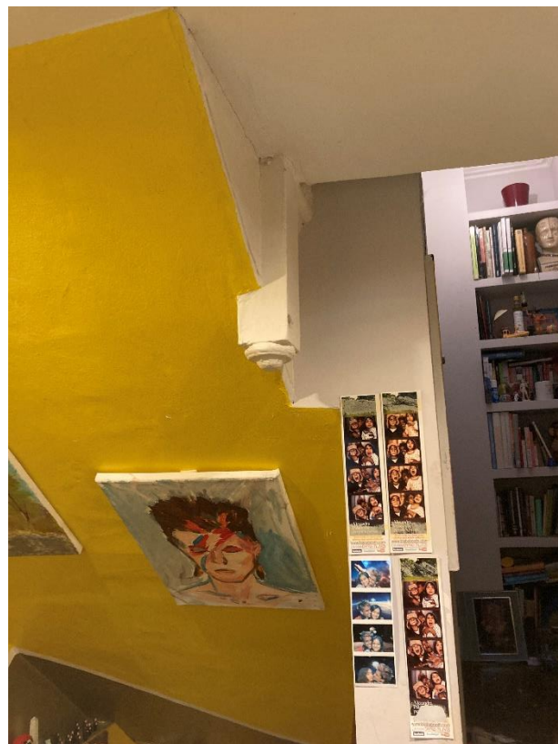
Figure 19: Newel Post, Ground to Lower Ground Halfway Landing
