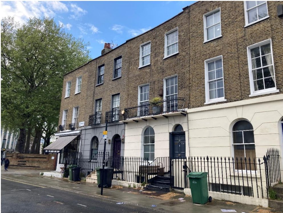
Figure 33: Nos. 132-126 St Pancras Way (right to left)
