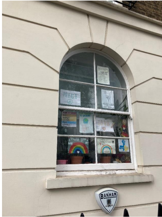
Figure 15: Semi-Circular Headed Window with Fluted Pilasters and Unoriginal Glazing Bars
