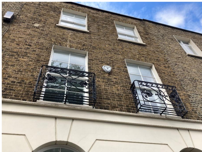
Figure 16: Decorative Iron Balconies
