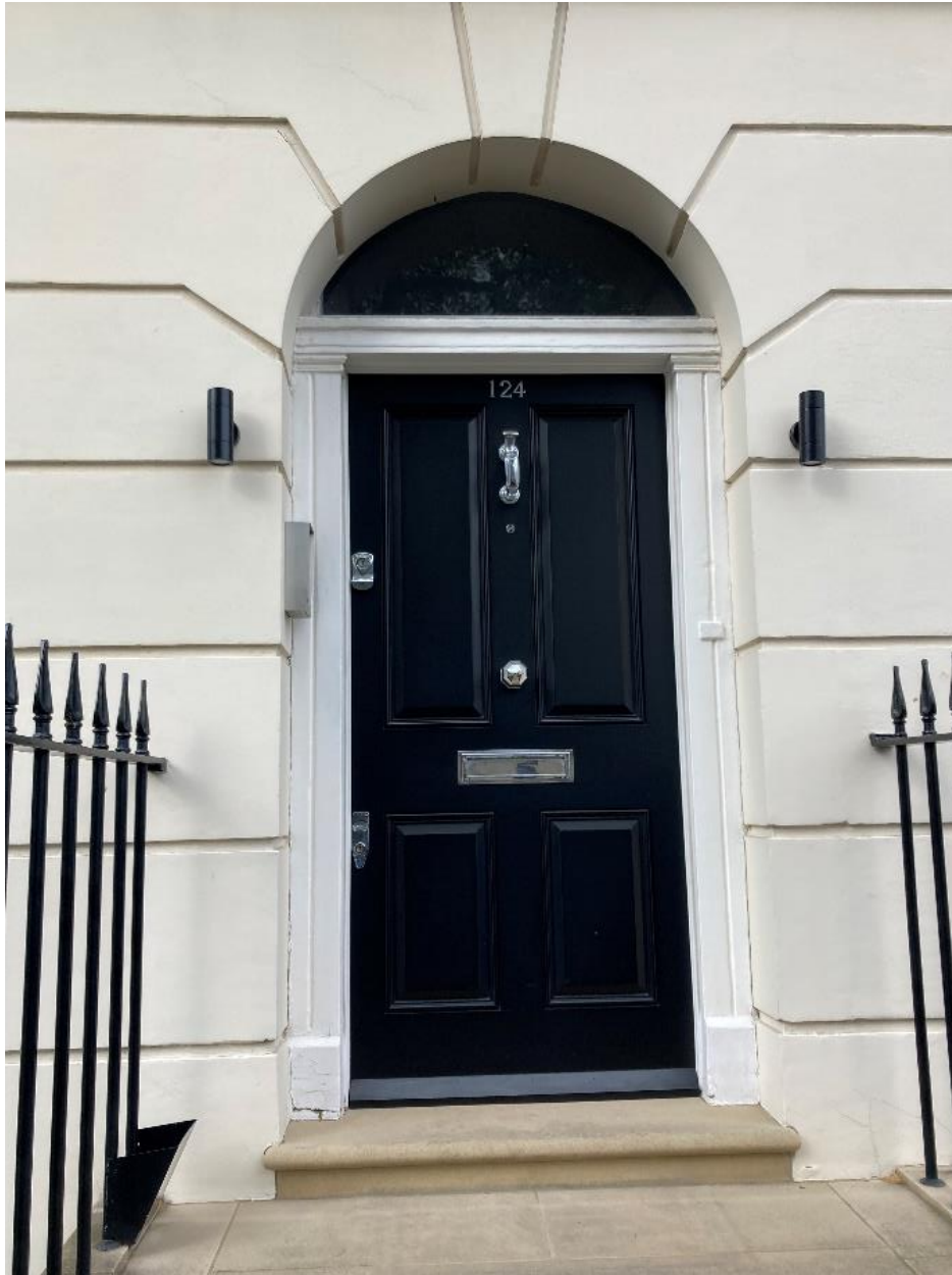
Figure 17: Entrance doorway with fluted pilasters, a semi-circular transom light, and sympathetically replaced four panelled door
