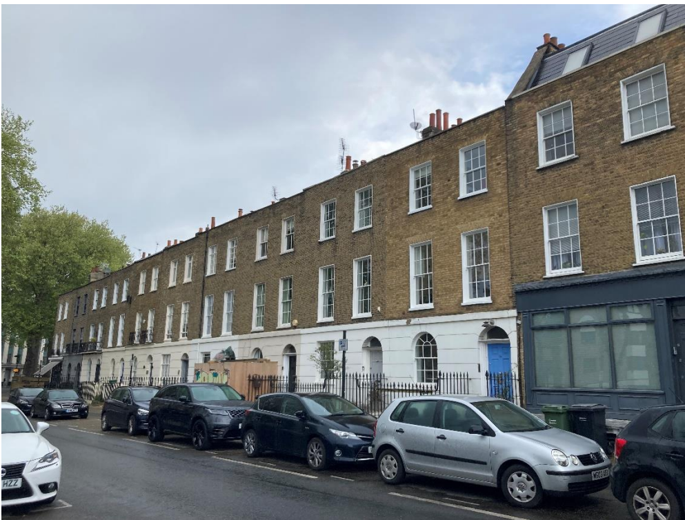
Figure 34: Nos. 132-122 St Pancras Way (right to left)
