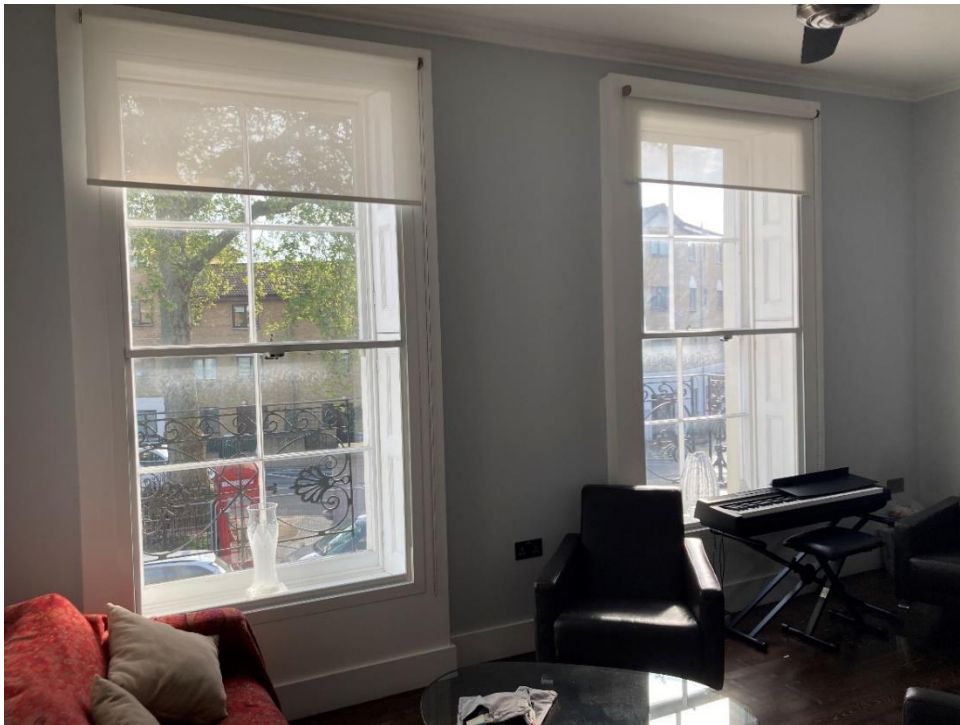
Figure 26: First Floor Windows with Original Shutters and Approved Secondary Glazing Boxing
