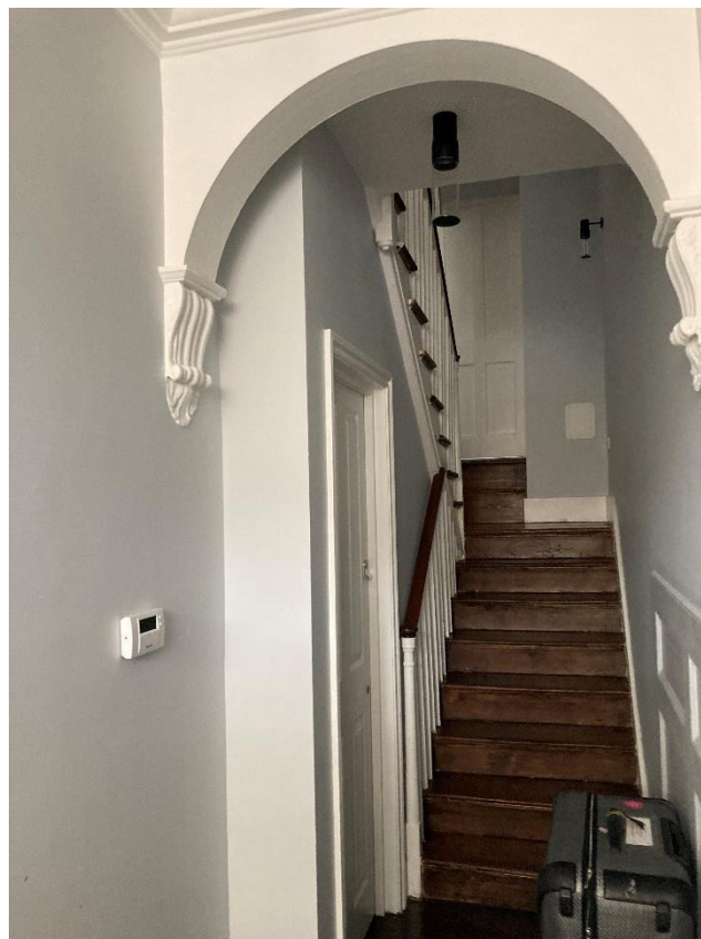
Figure 24: Console Bracket and Corresponding Archway to Ground Floor Hallway
