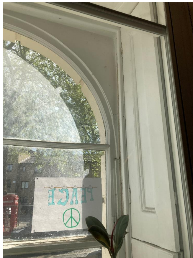
Figure 20: Ground Floor Front Room's Original Window Shutters Behind Secondary Glazing
