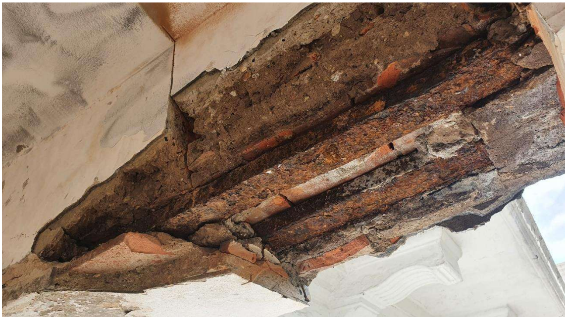
Figure 20 - Opened up Portico to the underside of a beam
