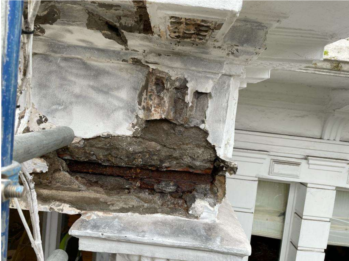
Figure 19 - Opened up Portico at the end column
